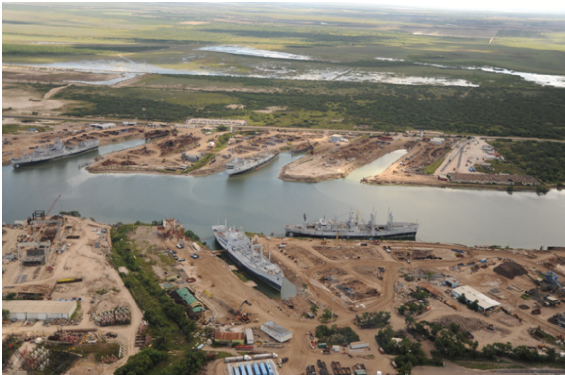
Figure 2.2 – Facilities Along Brownsville, TX, Ship Channel
