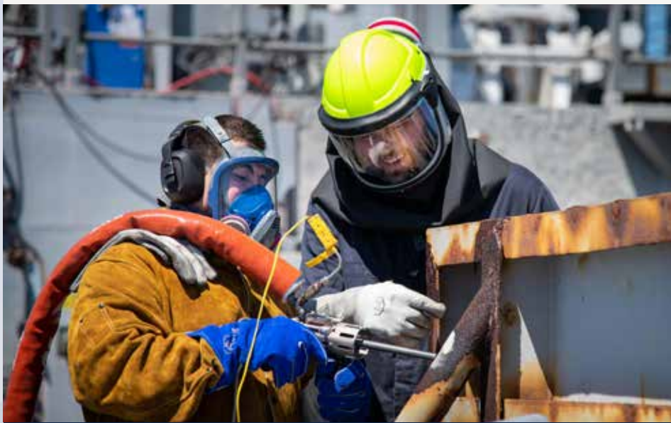
Surge Maintenance Hull Maintenance Technician 2nd Class Gerardo Vasquez (left) tries out for the first time the Dragonfly cold spray system with a hand spray applicator under the guidance of VRC Metal Systems Cold Spray Technician Ben Richard (right) aboard the Self Defense Test Ship (U.S. Navy photo by Eric Parsons)
