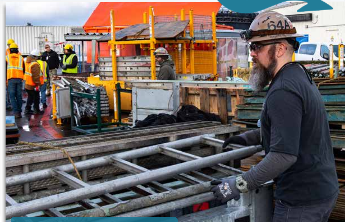
A TRFB team member works at Delta Pier.
