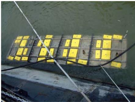
*Large four section patch assembly on the surface.*
