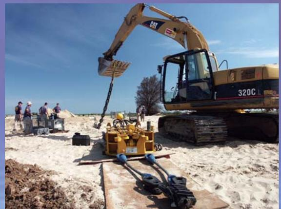
*MDSU-1, Det 1 works to set up beach gear to assist refloating of T/V STATE OF MAINE.*
