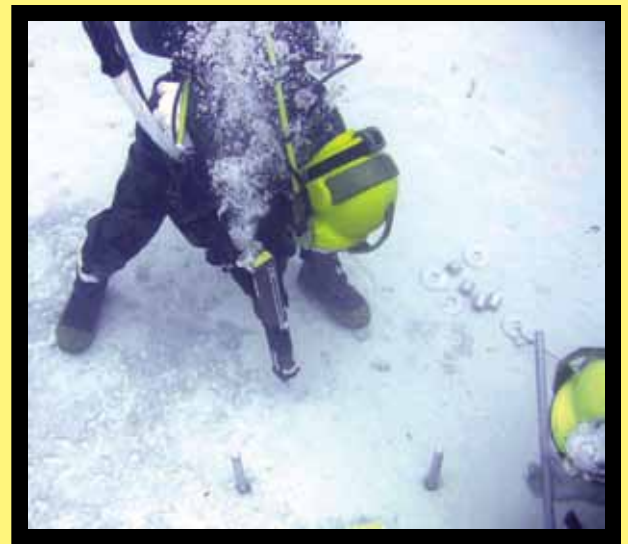
BU1(SCW/DV) Brian Strantz and EA1 (SCW/DV) Wyatt Boettger mount all-thread bolts to the sea floor with epoxy-grout using a pneumatic assisted dispenser. Photo by Jason Tanaka, NFESC.
