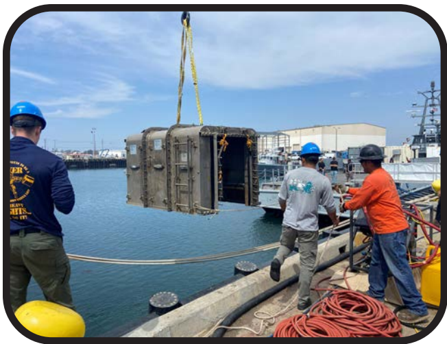
ND1 Scott Johnson directs installation of the dog-house cofferdam on the Ex-USS Paul Foster.
