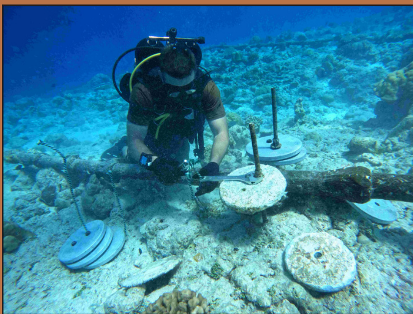
SW2 Andrew Cuellar installs new sacrificial zinc anodes on the Hydroacoustic Data Acquisition System (HDAS) to prolong the system's lifecycle.
