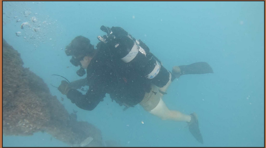
SW2 Andrew Cuellar installs new sacrificial zinc anodes on the Hydroacoustic Data Acquisition System (HDAS) to prolong the system’s lifecycle.
