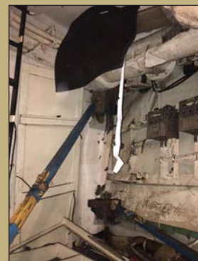
Salvage patching of bulkhead between Berthings 5 and 7 to make watertight and dewater Berthing 7.
