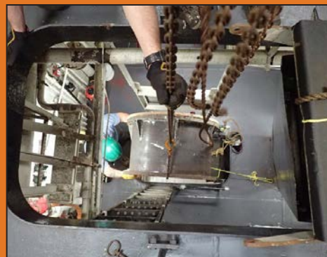
MCP Pipe-Flange Assembly Rigged into MER2.
