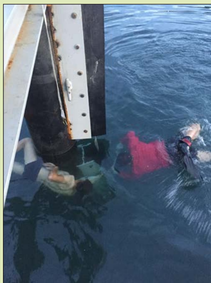
U.S. Navy Construction Mechanic 1st Class Matt Ramirez and Constructionman Adam Porras, both assigned to Underwater Construction Team 2's Construction Diving Detachment Bravo, attach fender system components to a pier in Dili, Timor-Leste on March 22, 2018. (U.S. Navy photo by Construction Mechanic 2nd Class Robert Norton)
