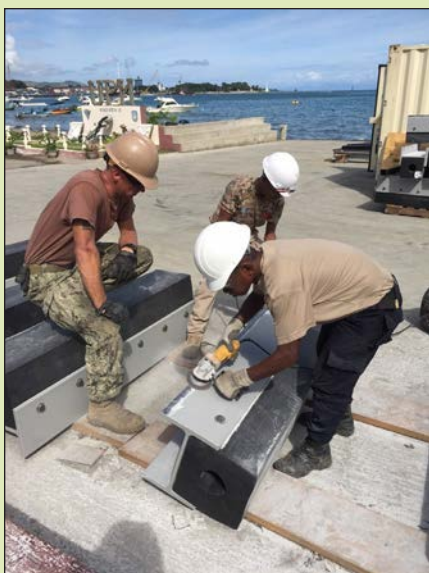
U.S. Navy Construction Mechanic 2nd Class Robert Norton, assigned to Underwater Construction Team (UCT) 2, works alongside Timor-Leste Maritime Police Unit Agents preparing fender system components that will be welded to a new pier in Dili Harbor, Timor Leste on March 9, 2018. (U.S. Navy photo by Lt. Michael Roster)
