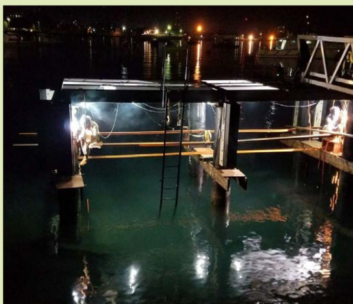
U.S. Navy Seabees assigned to Underwater Construction Team 2, Construction Diving Detachment Bravo (CDDDB) weld small boat fendering systems to the pile supported pier in Dili, Timor-Leste on March 23, 2018. (U.S. Navy photo by Lt. Michael Roster)
