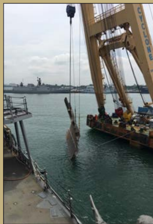
Patch being lifted into position.
