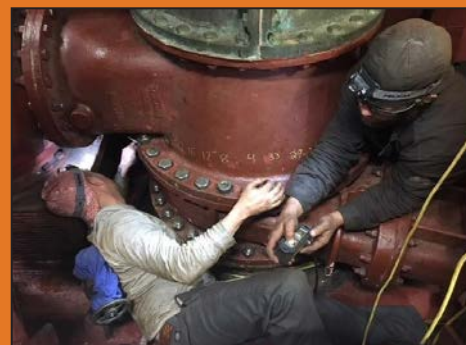
MCP Gate Valve Bolt Torque in MER2.
