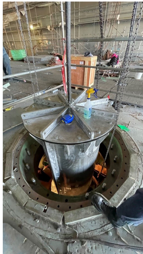
10ft tall top hat cofferdam extending above well deck. Photo by UWSH Division.
