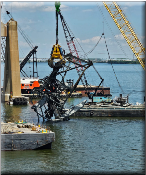
Salvage Wreck Grab and Chesapeake 1000 removing Key Bridge wreckage from the Patapsco River.
