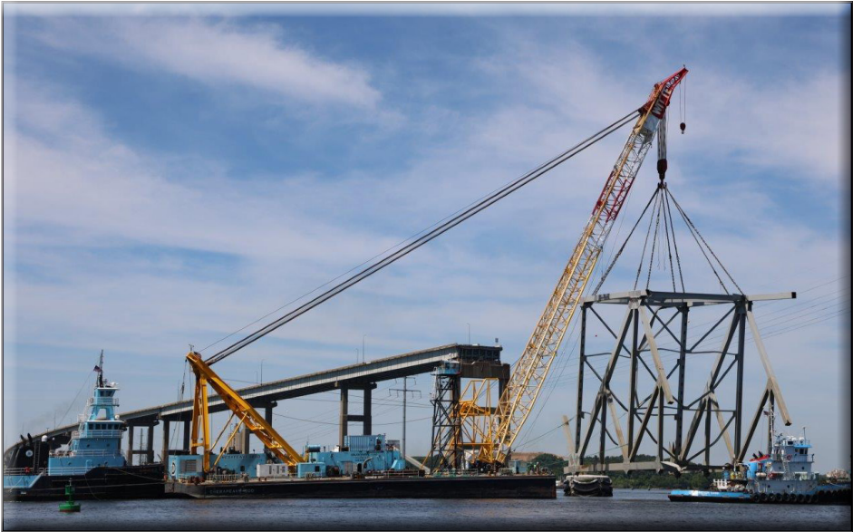
Chesapeake 1000 with 600 tons of truss in the hook - transiting to material processing yard.
