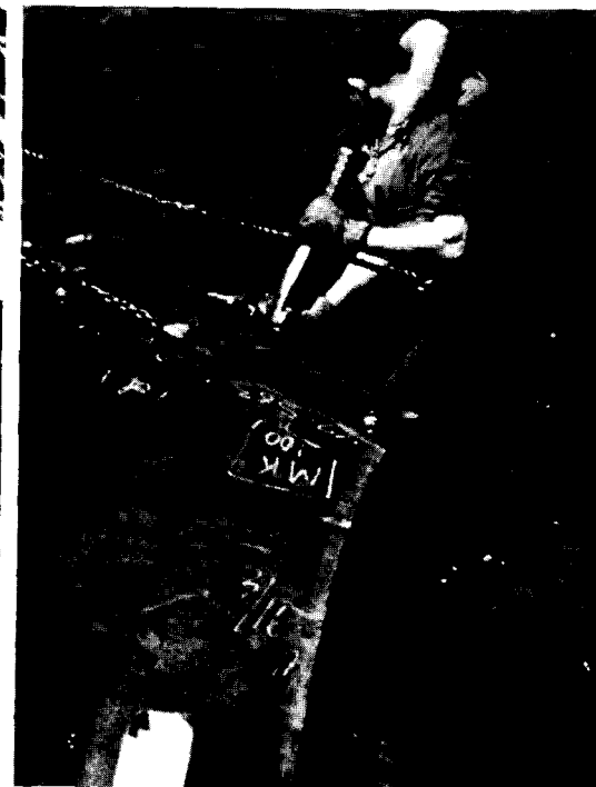
HTC John Bishop positions steel plate topside on bow of boat.
