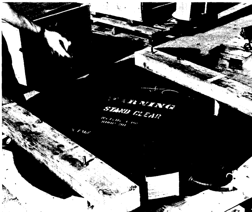
Divers uncrate the pilgrim nut backing plate.
