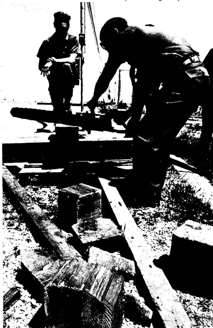
Divers practice using the hydraulic saw.
