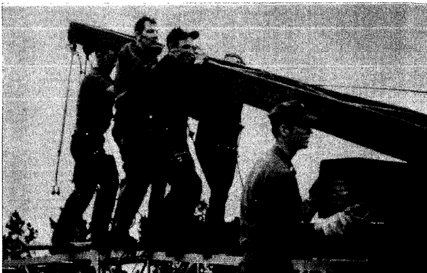
Newly assembled crane is raised into place by CBU 410 personnel.
