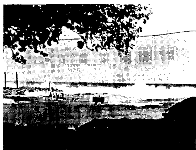
Work throughout the evolution was greatly affected by surf/current conditions. The concrete Dolphin located in the center of the photograph was explosively removed to allow the LCU to be turned in the harbor basin.
