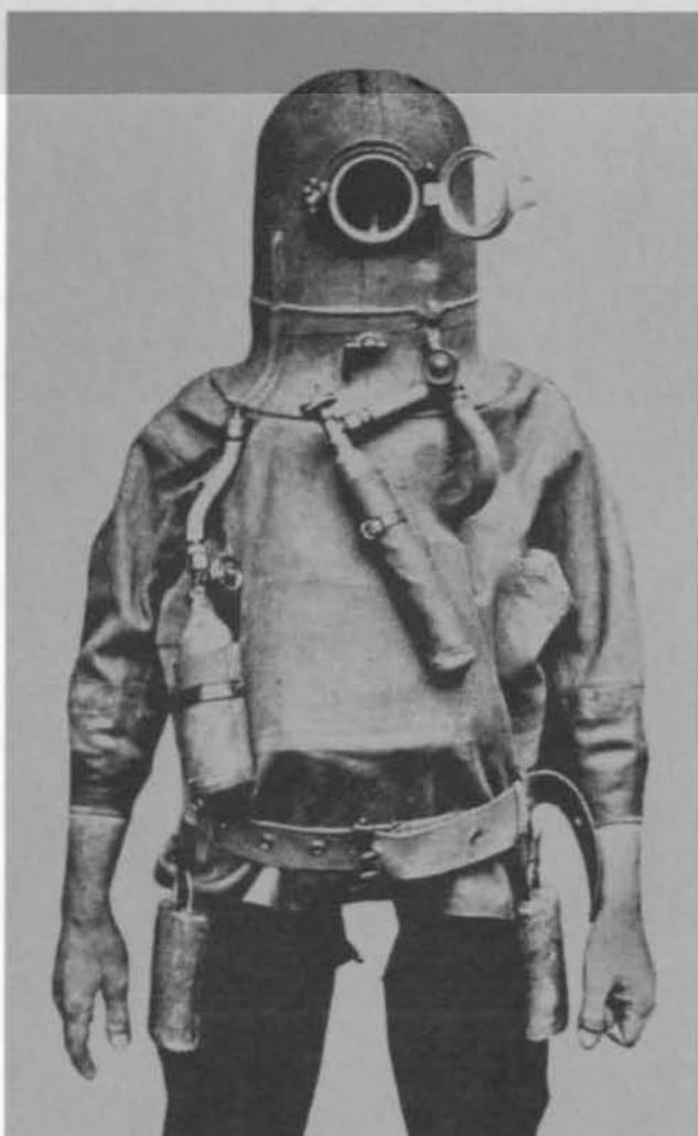
The Seibe-Gorman apparatus of 1914 (above) was a forerunner of today's Steinke Hood (right), which was developed at the Escape Training Tank in 1960. Buoyant ascent technique is taught to all Submarine Service personnel.
