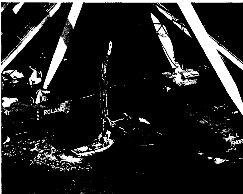
THOR and ROLAND parbuckle dredge 22 before lifting it.
