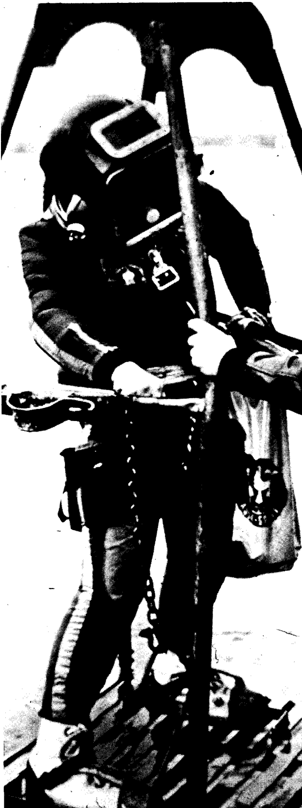
Diver suited in Mk XII is lowered by stage into water.
