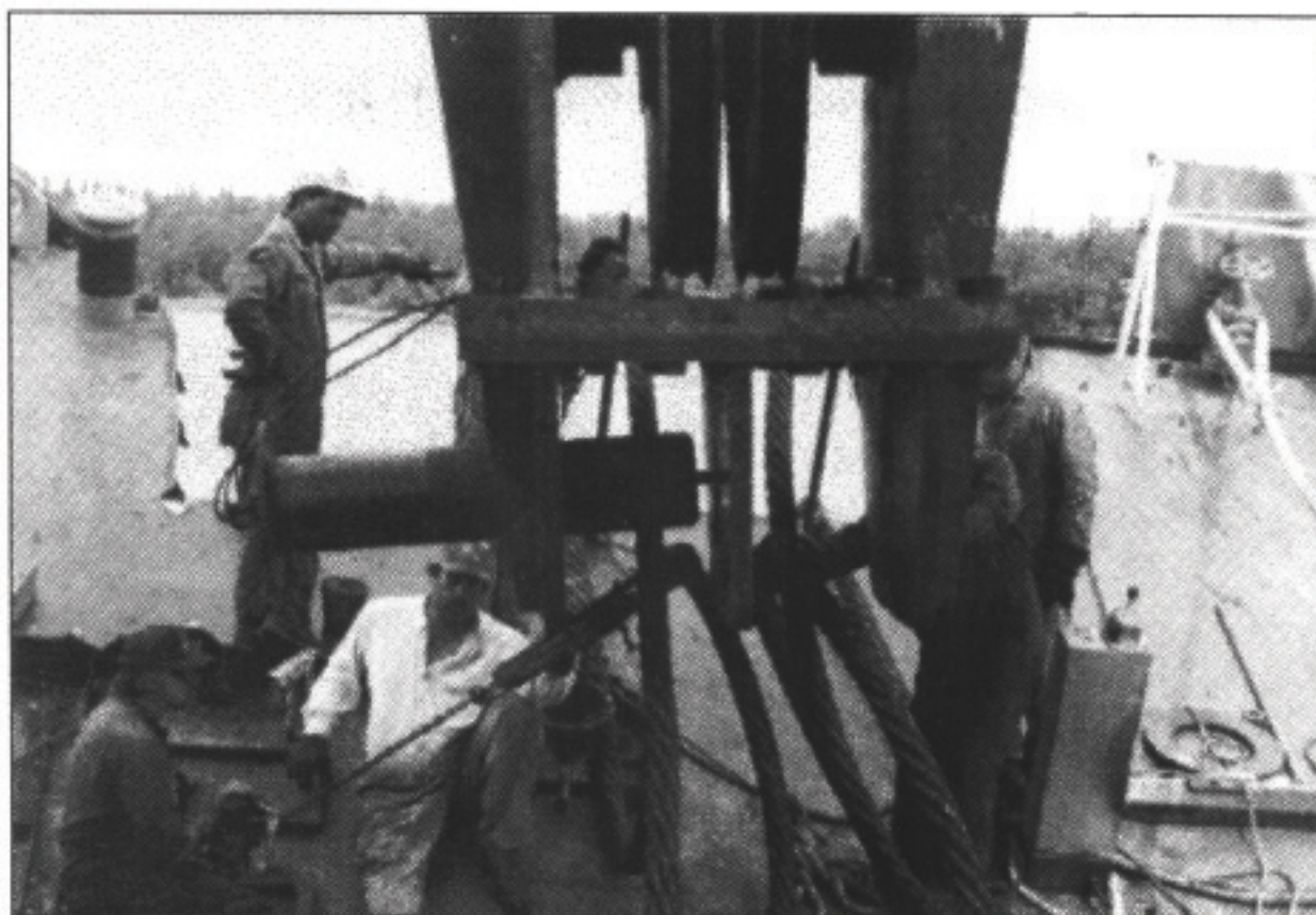
Figure 3-18. Lifting Pin Set to Capture Sling.
