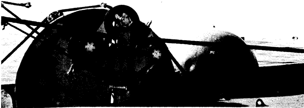
Photo # 16 Tensiometers Being Installed on Legs
