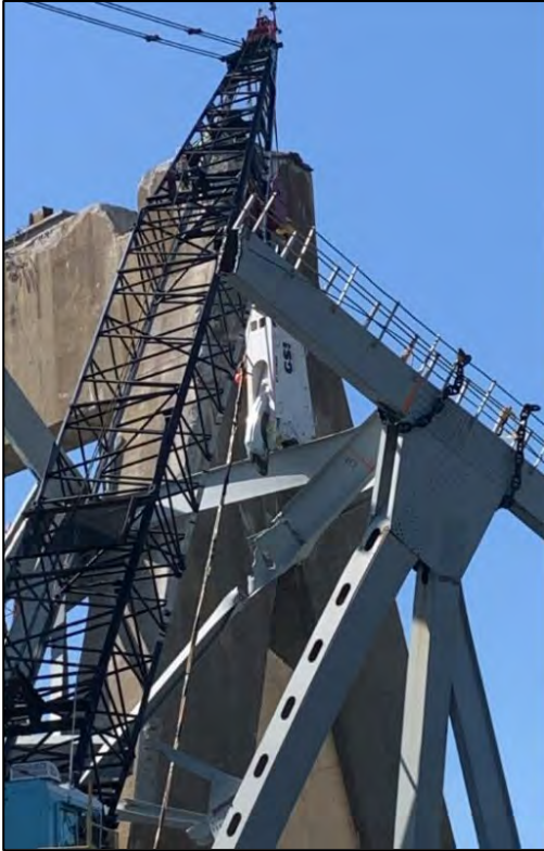
Figure 7-11 Crane barge Farrell's cutting shears used to separate truss 0 from the entanglements of the truss in span 19.
