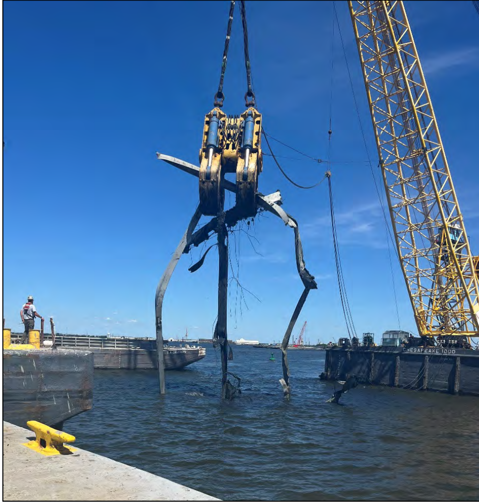
Figure 9-3 June 8: An example of steel debris still on the riverbed collected by CHESAPEAKE 1000 and the wreck grab.
