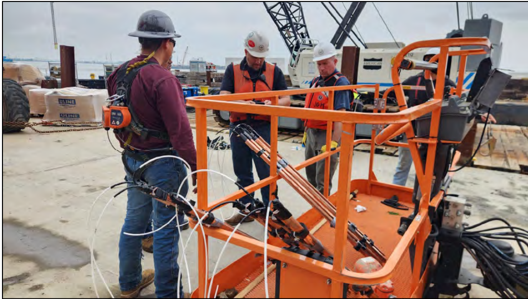
Figure 7-26 Shaped charges loaded onto manlift basket for placement at specified cuts.
