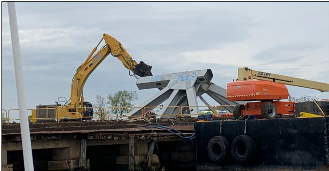
Figure 6-3 April 21: Skanska scrapping yard at work on a section of truss.
