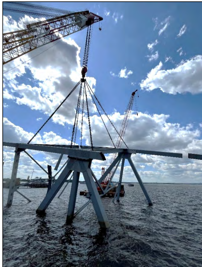
Figure 7-42 May 31: CHESAPEAKE 1000 lifting section 4-B breaking mud suction and determining what connections remained that required severing.
