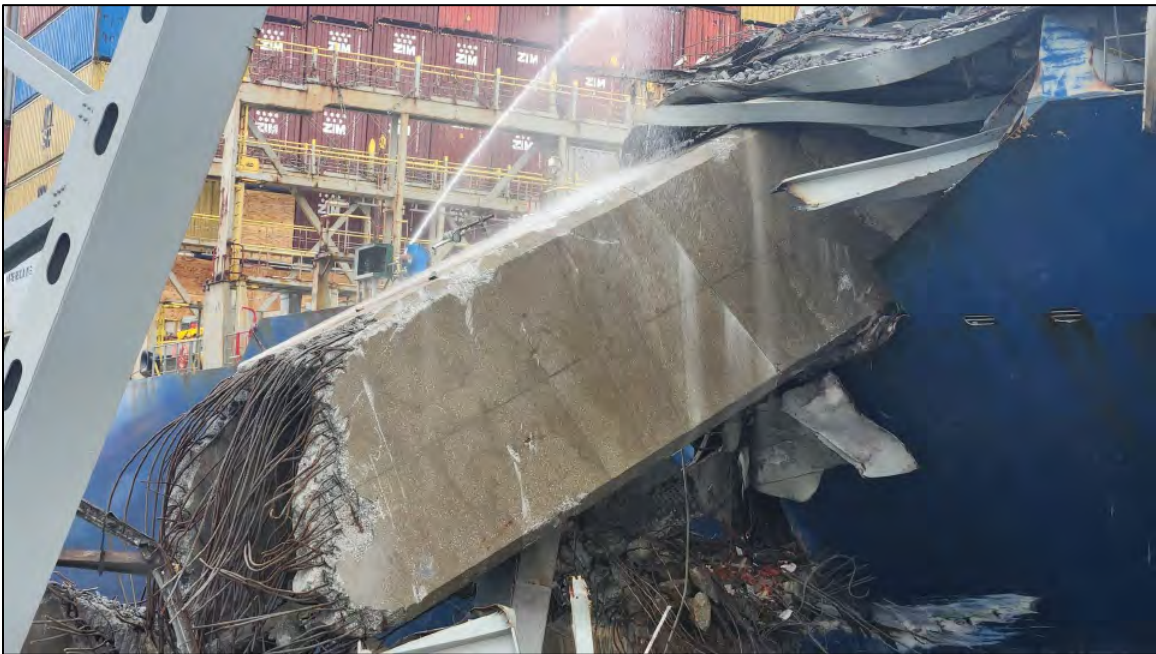
Figure 7-20 Concrete pillar cutting using a diamond wire saw.
