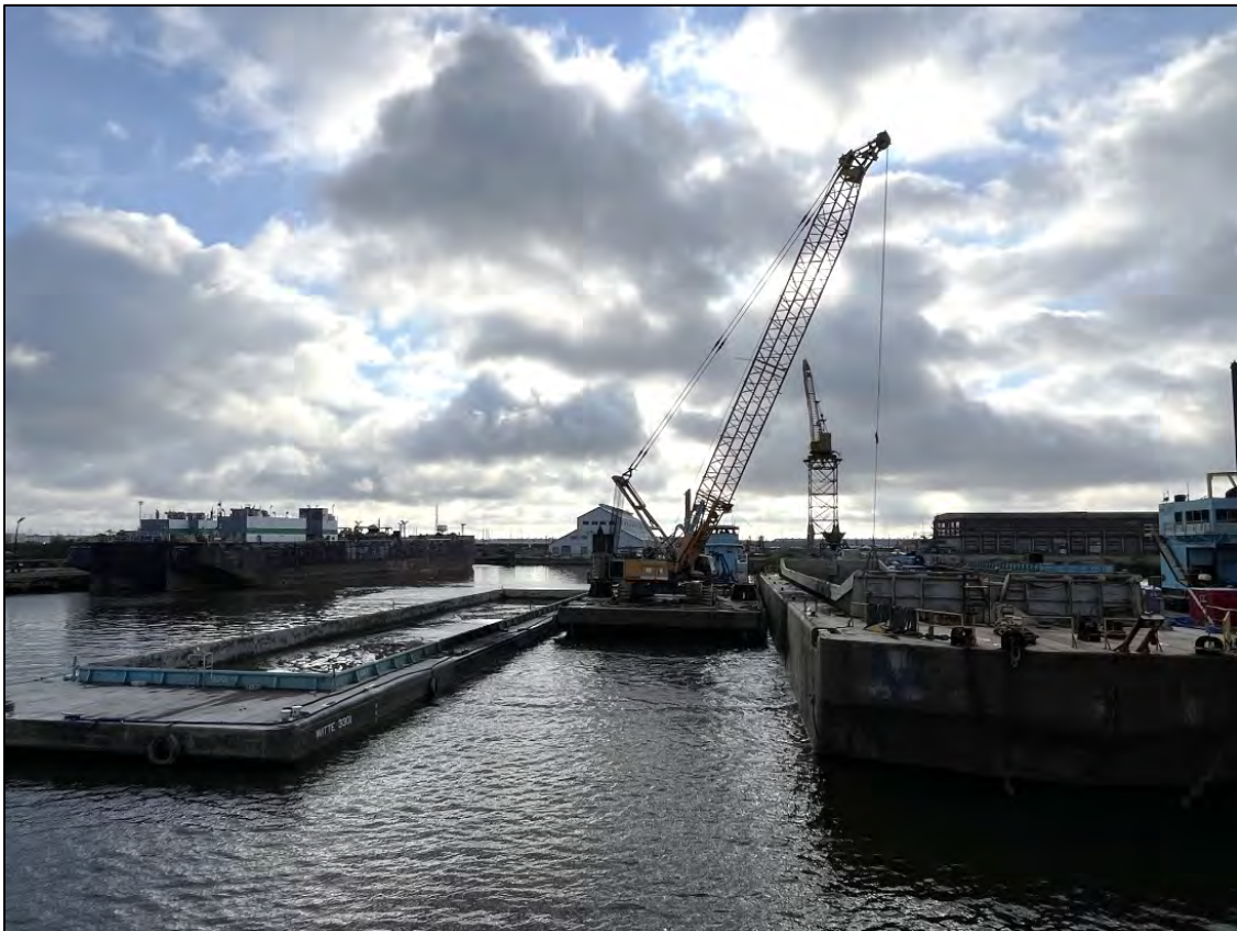
Figure 8-1 Transloading displaced material pierside between barges. River barge on left, ocean scow on the right. Mix of debris within the mud consisting of steel remnants and roadbed material.
