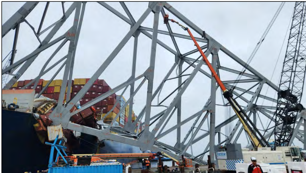
Figure 7-27 Charges being placed during the week of 6 May.
