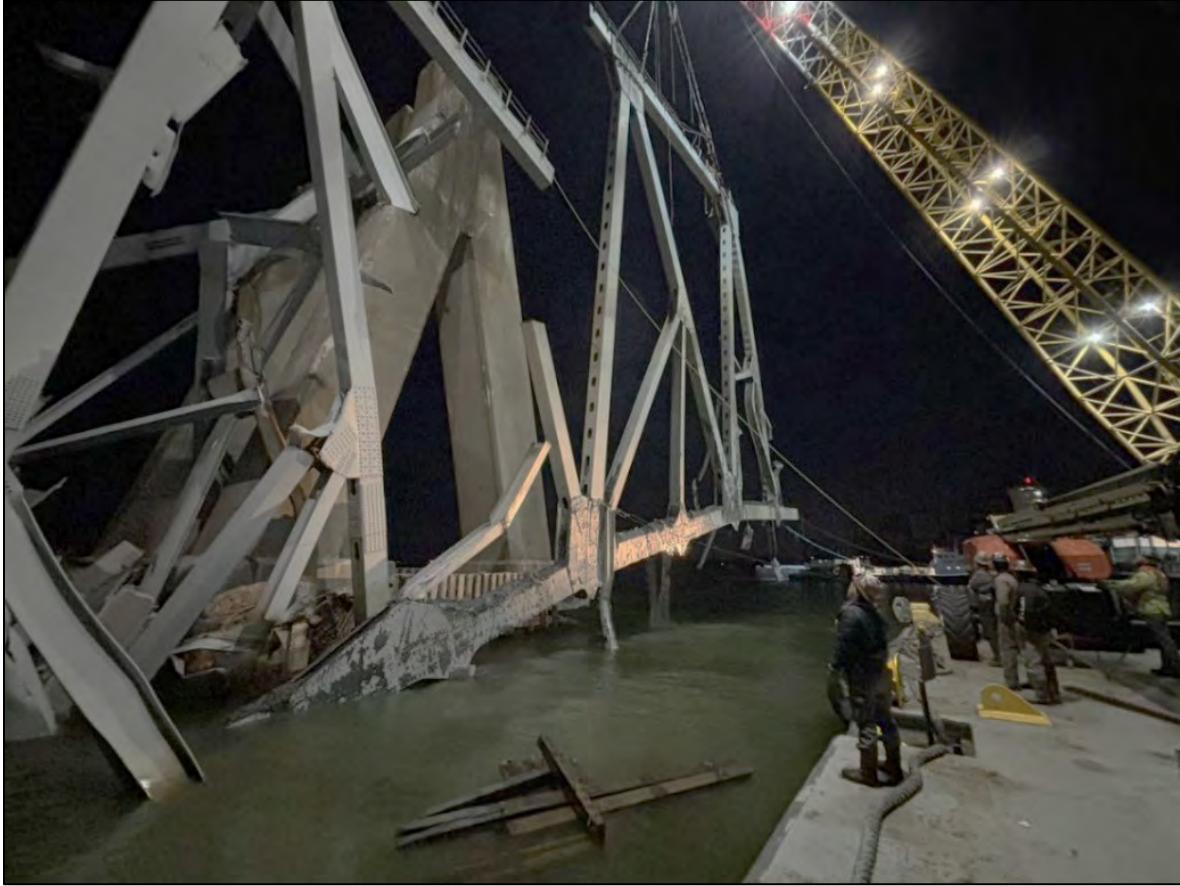
Figure 7-10 Truss section 0-B being pulled from the water at about 0130 on 23 April.
