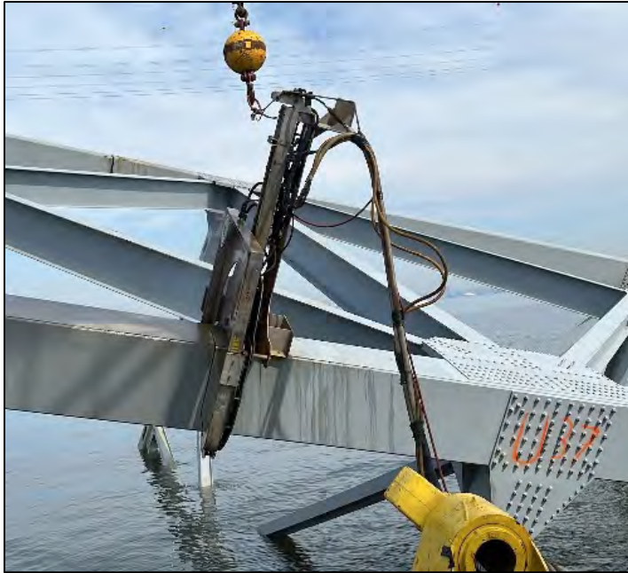
Figure 7-41 Diamond Wire Saw cut IVO frame U37.
