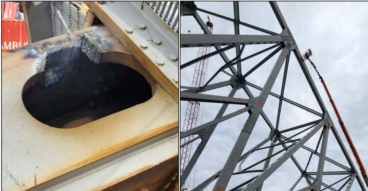
Figure 7-25 Left: Example of a “hot” pre-cut made in a truss member to allow effective placement of explosive charges. Right: Manlift hoisting welder to top of Truss 4 during pre-cutting operations.
