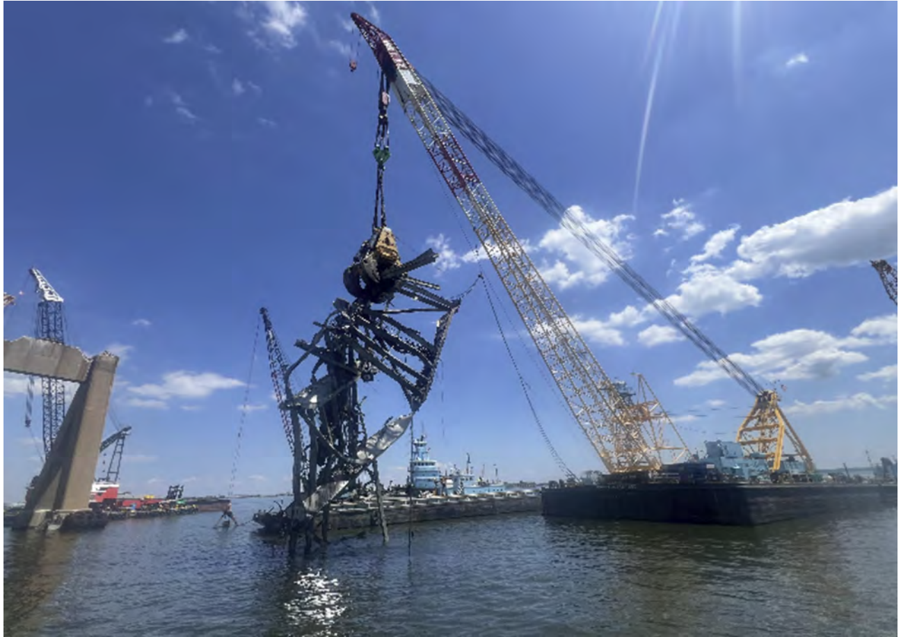
Figure 3 – Chesapeake 1000 with another large bridge piece lifted by “Gus” the 1000 ton grab.
