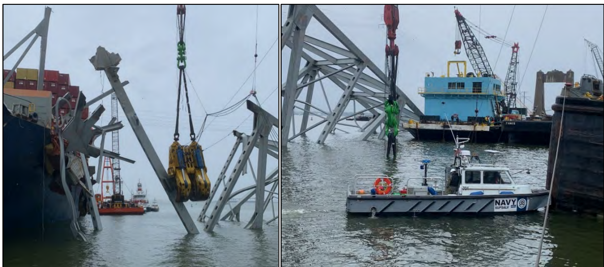
Figure 7-32 Left: the first hanger being collected by Donjon's wreck grab. The salvors found it was too long to clear the water's surface, so they lowered it back to the riverbed. Right: the wreck grab lowered to the bottom, attempting to find a better purchase on the truss section with the ESSM boat operators broadcasting the CODA Octopus picture "live" on Microsoft Teams, guiding the grab to the best location.
