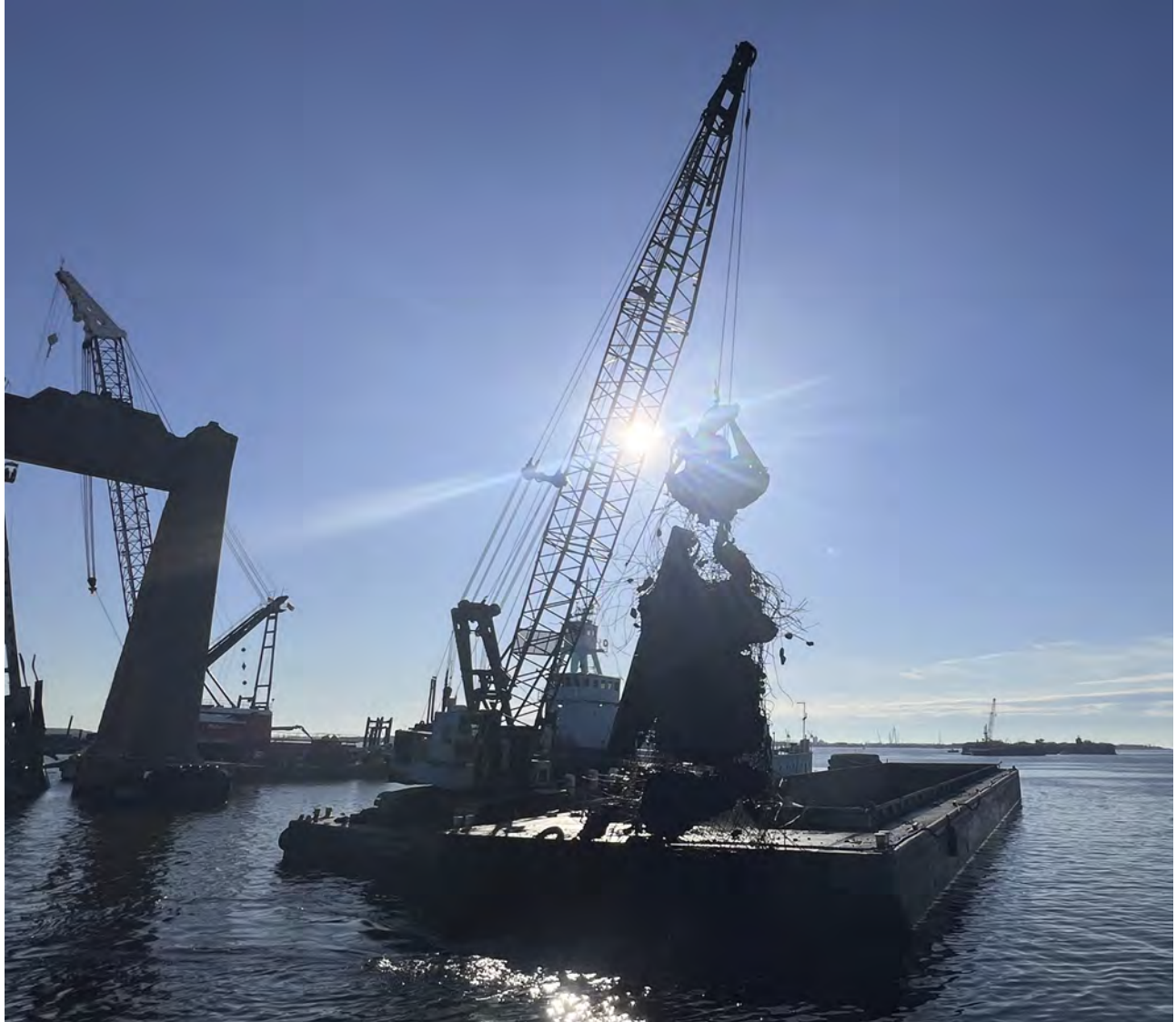
Figure 1 – Debris removal via bucket ops with dredge Oyster Bay transferring debris to Witte 3302 barge.
