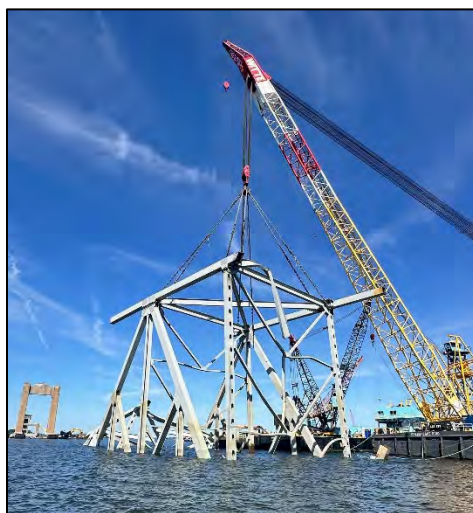
Figure 10-2 Roadbed material (rebar, concrete and steel) lifted from channel by OYSTER BAY.
