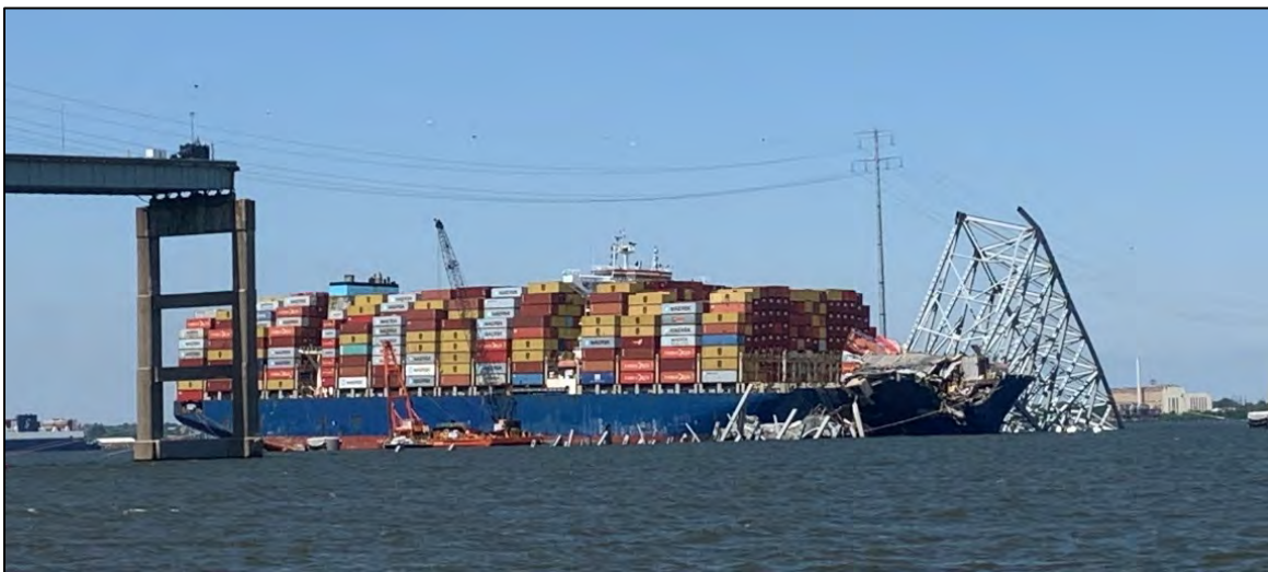
Figure 7-23 Truss 17 material remaining above the water at low tide after the teams made their lifts the week of 8 May.
