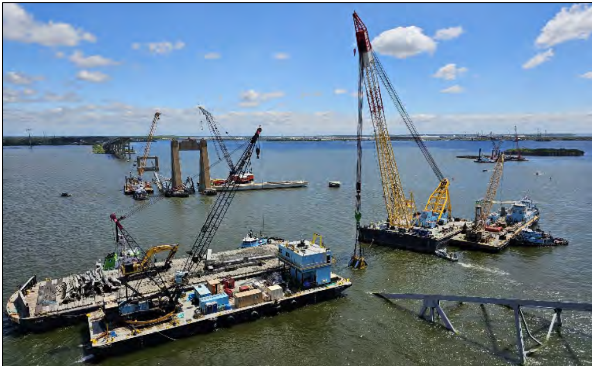
Figure 7-35 May 16: Donjon equipment clearing the riverbed at the foot of Section 4.
