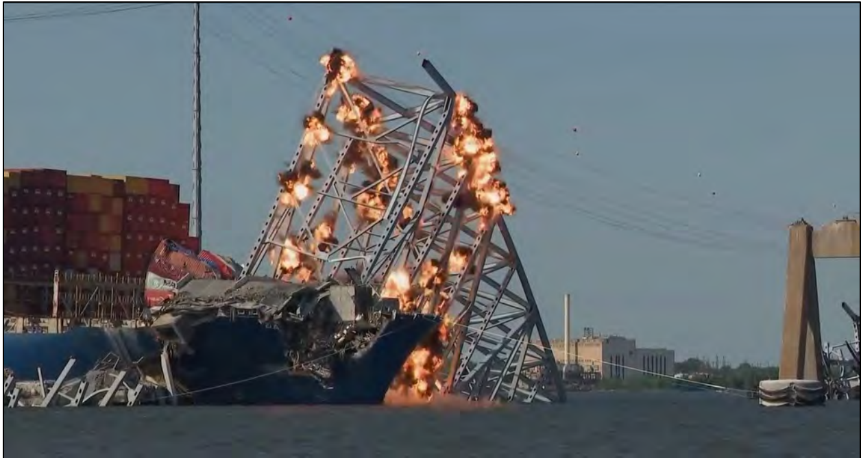
Figure 7-28 Section 4 Explosive Demolition.
