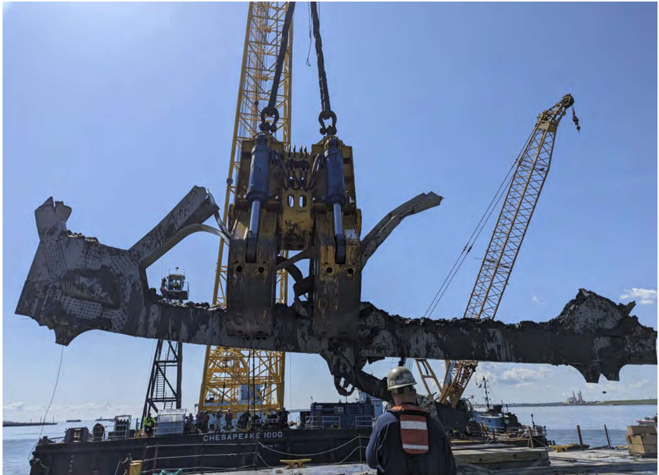
Figure 2 – Chesapeake 1000 lifts large bridge debris and transfers to material barge James.
