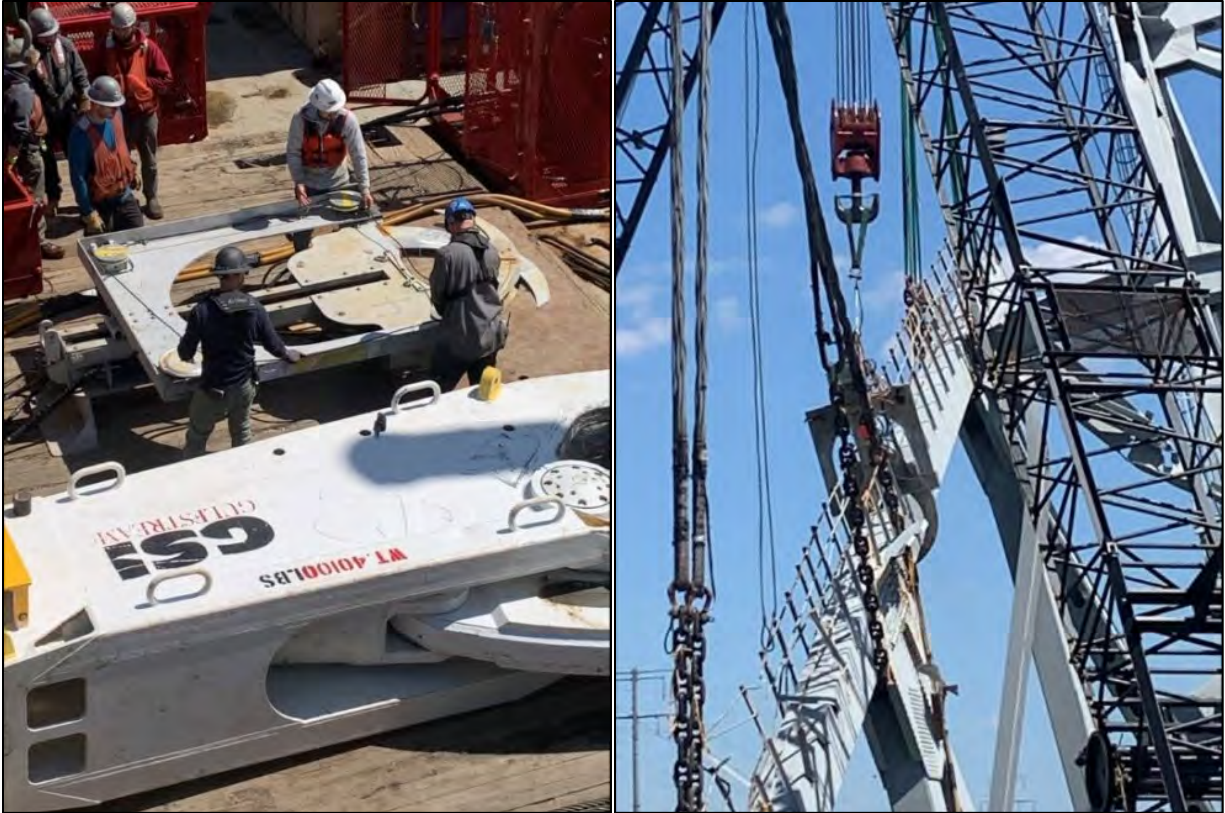
Figure 7-8 Left: Hydraulic cutting shears (foreground) and diamond wire saw on deck of the crane barge Farrell. Right: Diamond wire saw in use on the top cord of truss 0.
