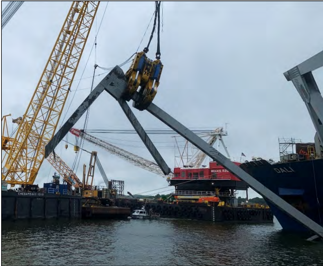
Figure 7-33 The same truss piece, after repositioning the grab. This was transported directly to the Skanska steel processing yard as it was too long to lower to the barge deck.
