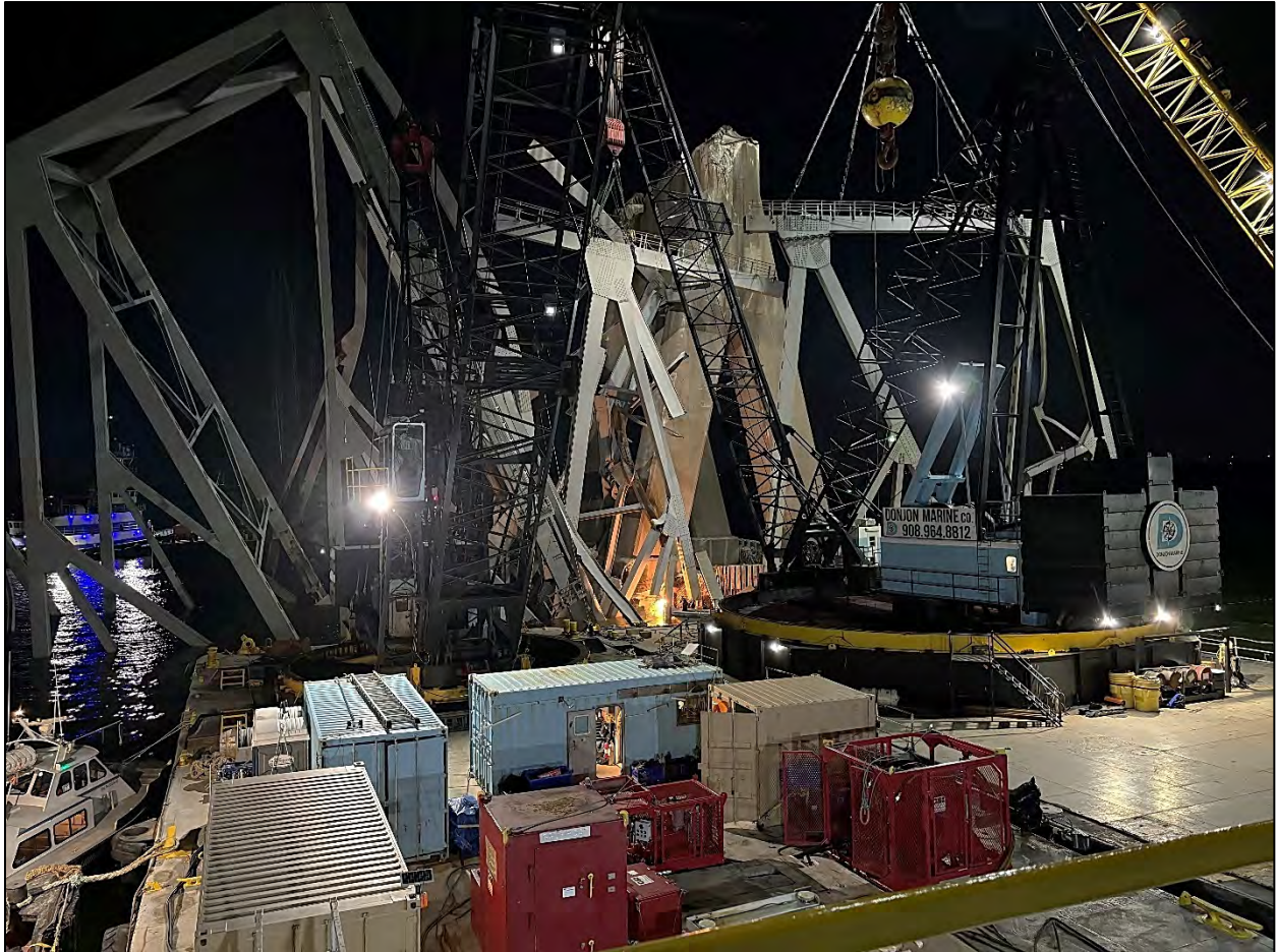
Figure 1-1 A challenging lift of 'Section 0' requiring multiple cranes and separation of structure by torch cutting.
