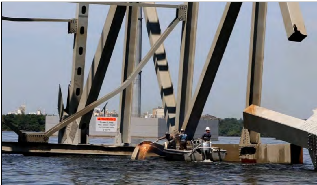
Figure 7-44 June 1: Torch work to clear remaining connections between Section 4-B from 4-C.
