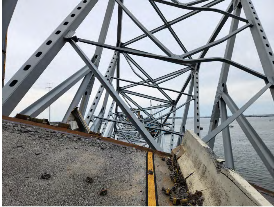
Figure 3-2 Buckled Lateral Support at Panel 29
