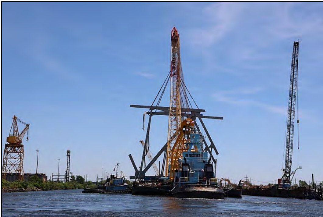
Figure 6-4 June 3: Donjon's CHESAPEAKE 1000 delivering section 4-B to the processing yard.
