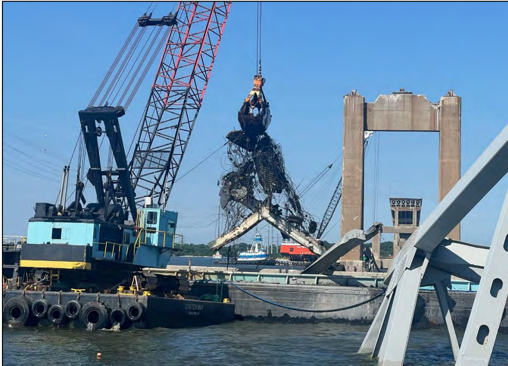
Figure 10-1 Section 4A being lifted from channel by CHESAPEAKE 1000.
