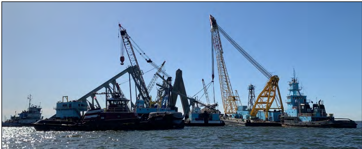
Figure 5-2 April 22: Donjon vessels working together on truss section 0.
