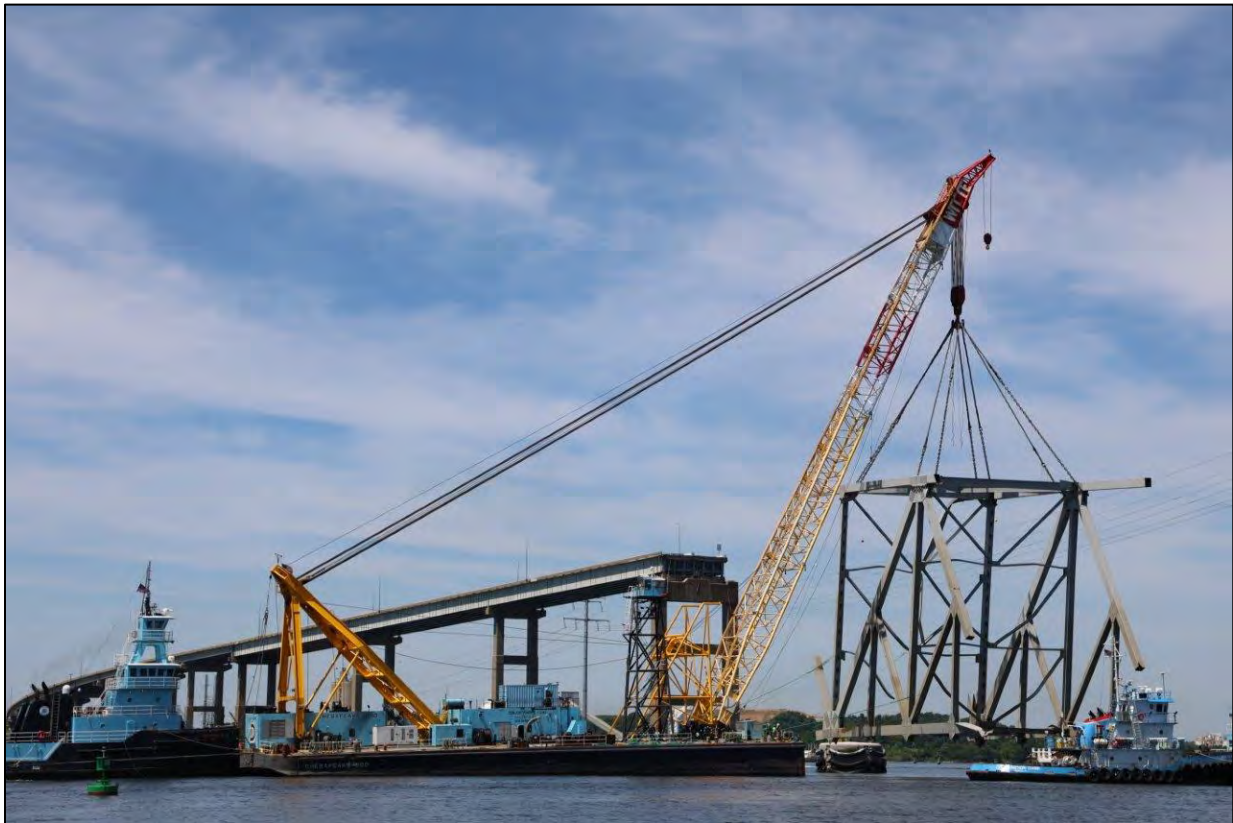
Figure 7-45 June 1: Section 4-B lifted and beginning transit back to Sparrows Point. This section of the bridge weighed in at 560 tons.
