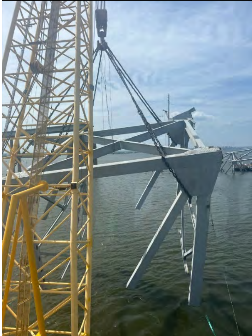
Figure 7-21 May 8: CHESAPEAKE 1000 lifting truss section 17A from the water. This was a joint Donjon-Skanska effort while Resolve was finishing preparations for demolition of Truss 4.
