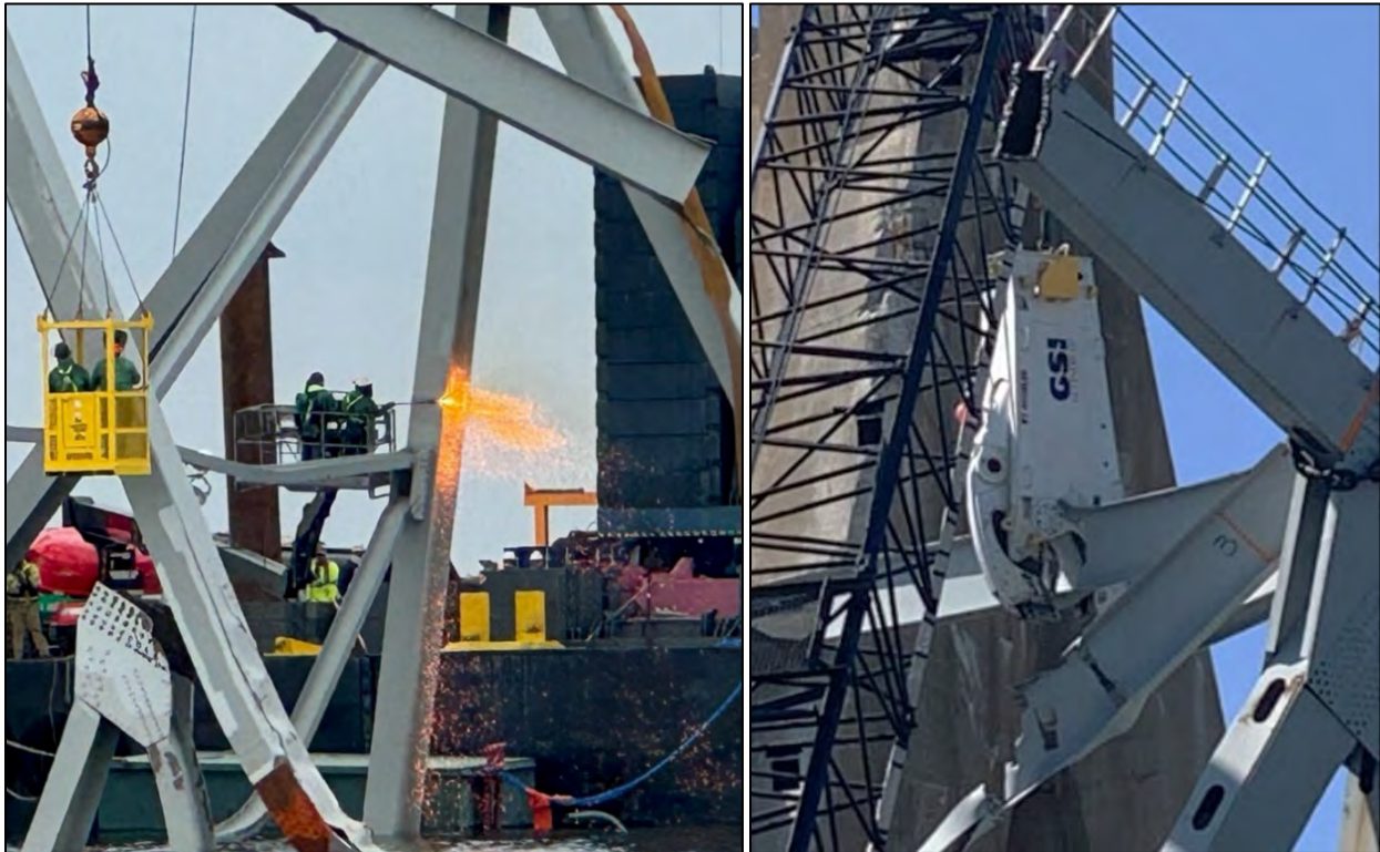
Figure 7-7 Truss cutting methods – torch work on left and hydraulic shears on the right.
