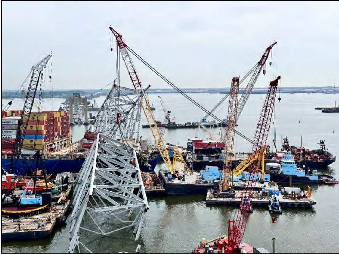
Figure 7-22 May 8: Skanska cranes (red) and Donjon cranes (light blue) work together to cut and lift truss section 17-1 just south of M/V DALI. This operation was the result of the two salvage companies joint planning and preparations.
