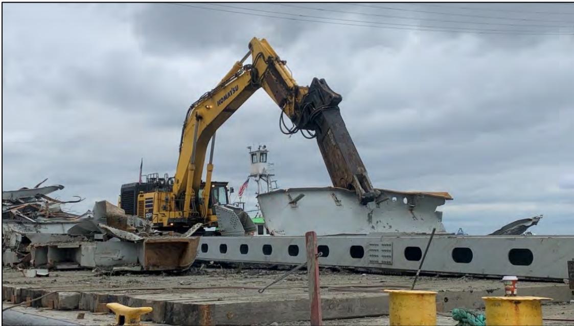
Figure 7-37 May 17: Deck crawler equipped with shears cutting and clearing steel deposited by the wreck grab.
