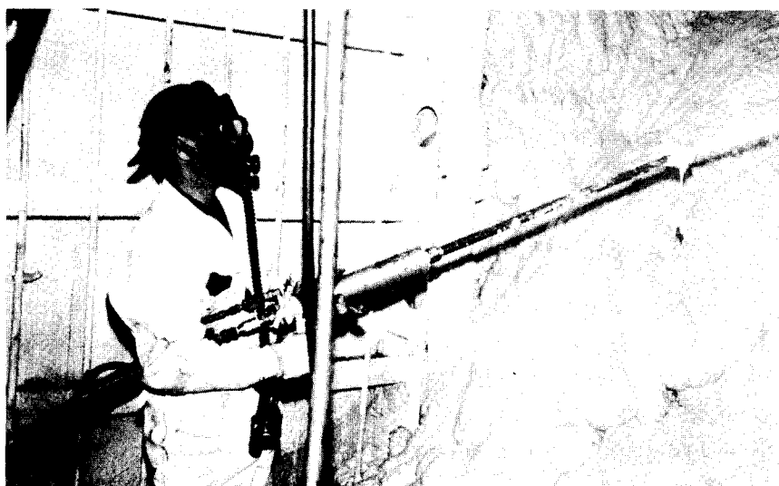
SRF Yokosuka workman is applying polyurethane to LST compartment with foam gun. Note supply hoses connecting gun to foam system set up on LST's tank deck. Breathing apparatus is necessary when applying foam in enclosed spaces, for protection against toxic fumes of the foam mix.
