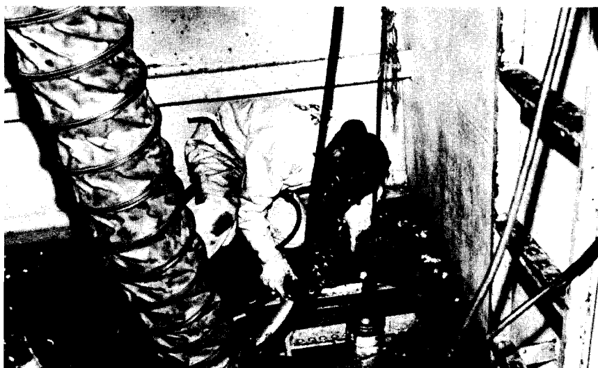
Foam gun is being directed through an access hatch as workman applies final amount of foam. Note blower supply duct used to reduce generated toxic fumes.
