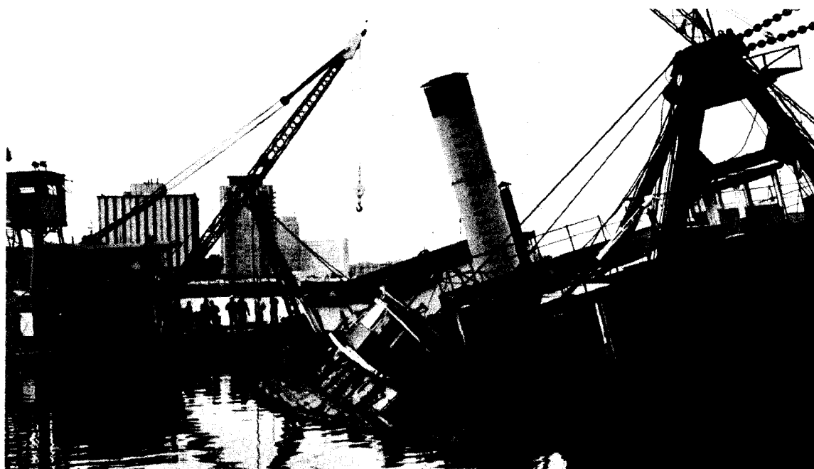
Oily water surrounds Dredge ATLANTIC and tug as salvors inspect casualty site aboard derrick barge YD-53. Top photo shows port side of dredge at high tide, looking forward; bottom photo is of starboard side at low tide, looking aft.
