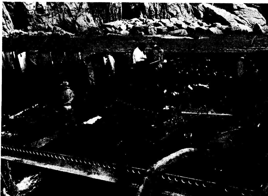
Diver prepares to leave diving station to conduct cutting operations. The stern section served as a diving station for transverse cutting of the hull at frame 106.5.
