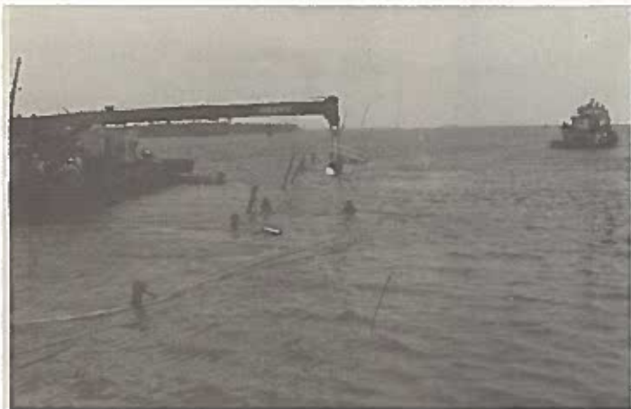
PHOTOGRAPH 38. Preparations nearing completion for dewatering of port side of forward section (Phase Three).
