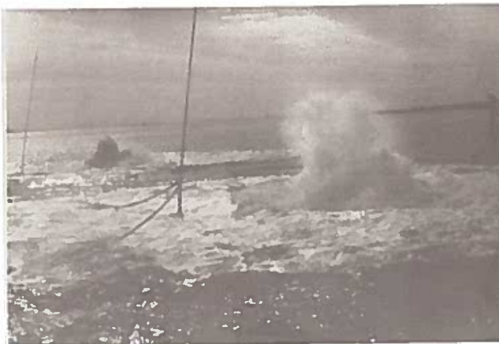
PHOTOGRAPH 31. Venting continues. Vertical poles were installed to provide initial indications of movement.
