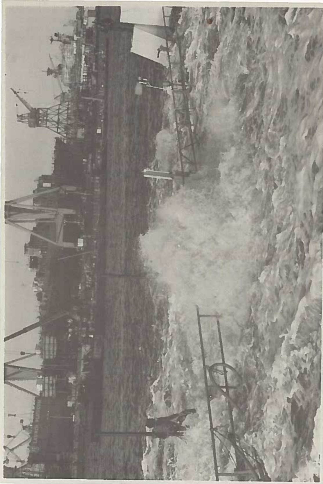
PHOTOGRAPH 11. Rupture on outboard wing wall which led to abortion of Phase One plan to blow with air. (Estimating the size of a leak by the size of the bubble is difficult. This spectacular boil was caused by an 8"x1" (max.) tear in a corner weld. The differential pressure across the rupture was only 15 FSW; it leaked at the rate of 1200-1800 SCFM. The air of course expanded rapidly during its free rise of 33 ft to the surface.)
