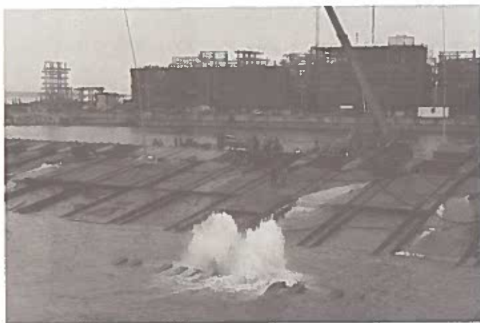
PHOTOGRAPH 43. Pontoon Deck begins to level as keel blocks become visible.
