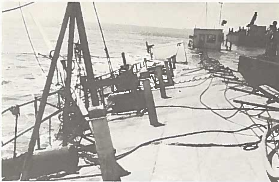
PHOTOGRAPH 22. Tugs continue pulling as port side continues to rise.
