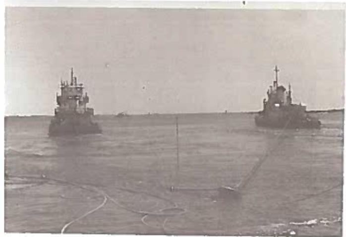
PHOTOGRAPH 15. Tugs made fast to port side capstan to snake section from beneath control house overhang of forward section.
