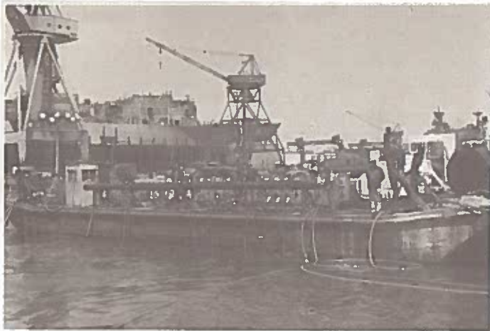
PHOTOGRAPH 14. Control barge being readied for Phase Two dewatering attempt on port side of aft section.
