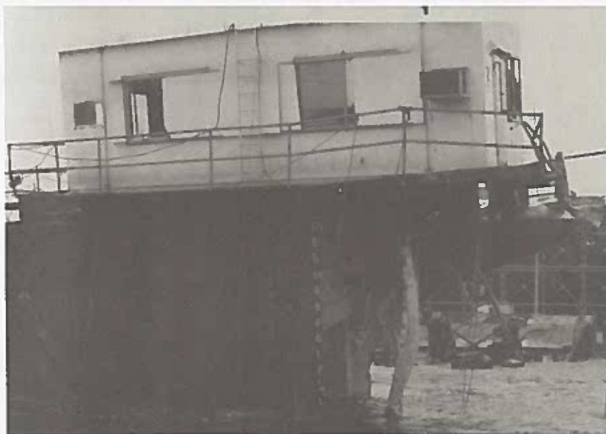
PHOTOGRAPH 45. Underwater oxy-arc cutting performed by divers beneath control house to facilitate snaking of aft section from beneath.
