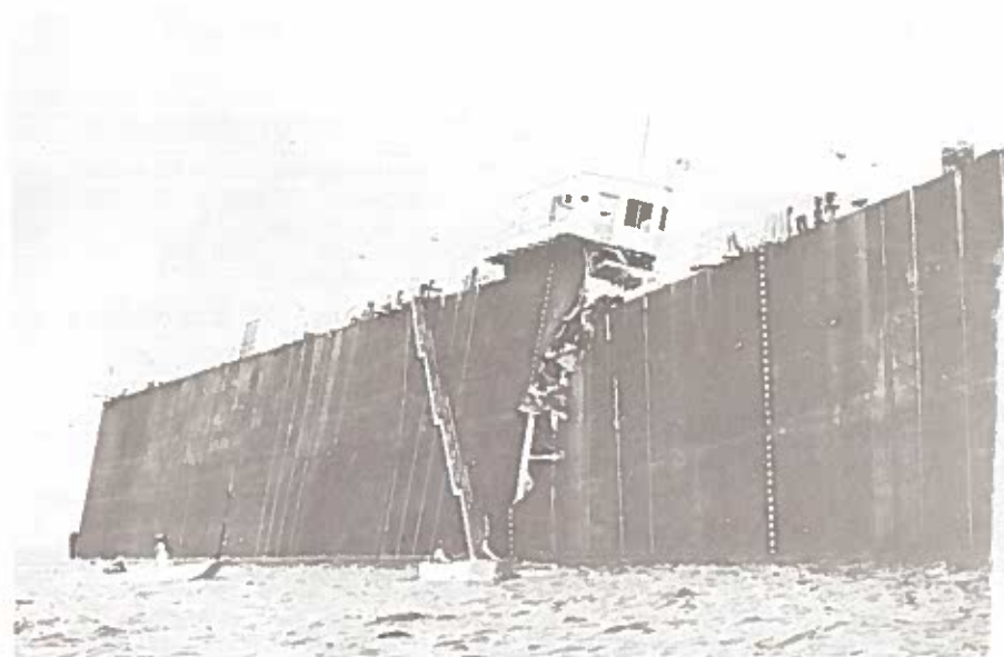
PHOTOGRAPH 4. Launching platform failing amidships in combined shear and compressive buckling.
