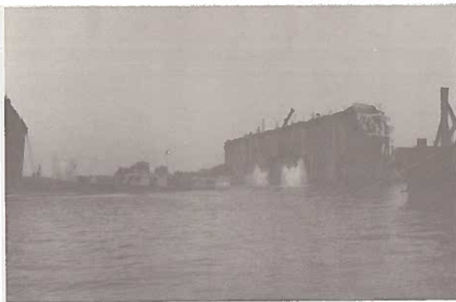
PHOTOGRAPH 25. Aft section dewatering continues. Entire Pontoon Deck almost awash.
