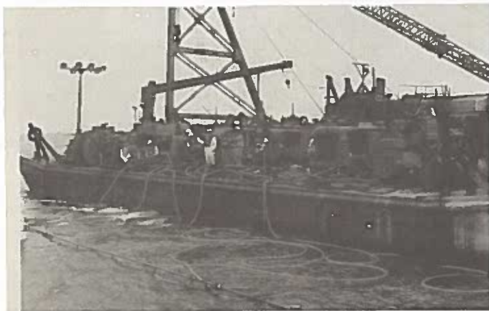
PHOTOGRAPH 7. Control barge outfitted with air compressors and manifold connected to launching platform air vents.
