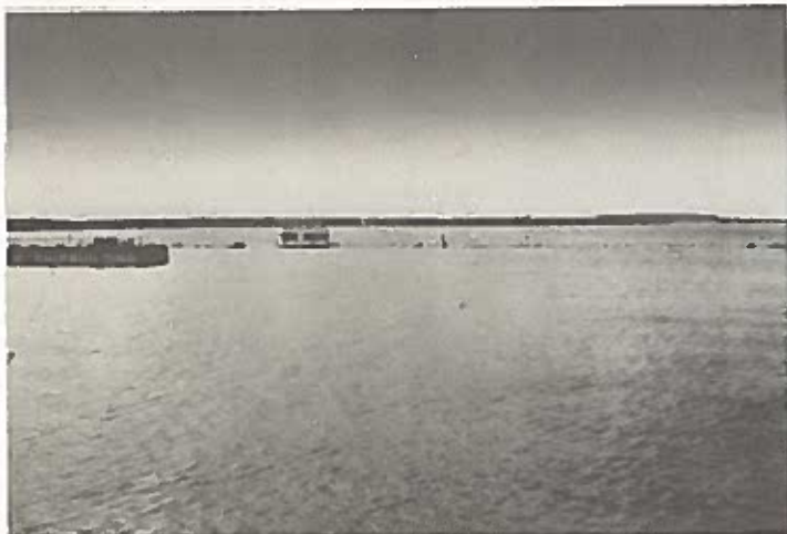
PHOTOGRAPH 5. Launching platform resting on the bottom in 72 ft. of water.
