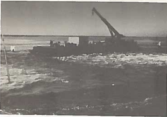
PHOTOGRAPH 33. Pontoon Deck breaks the surface. Forty-eight foot ascent required approximately one minute.
