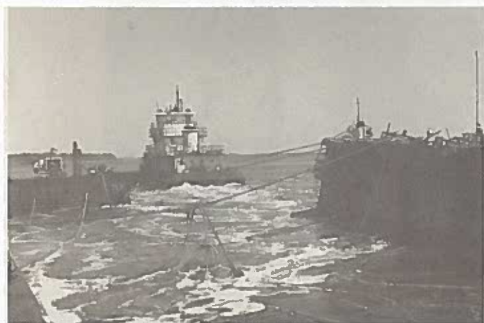
PHOTOGRAPH 19. Tugs continue pulling aft as aft end of platform section continues up with forward port corner still embedded in bottom mud.
