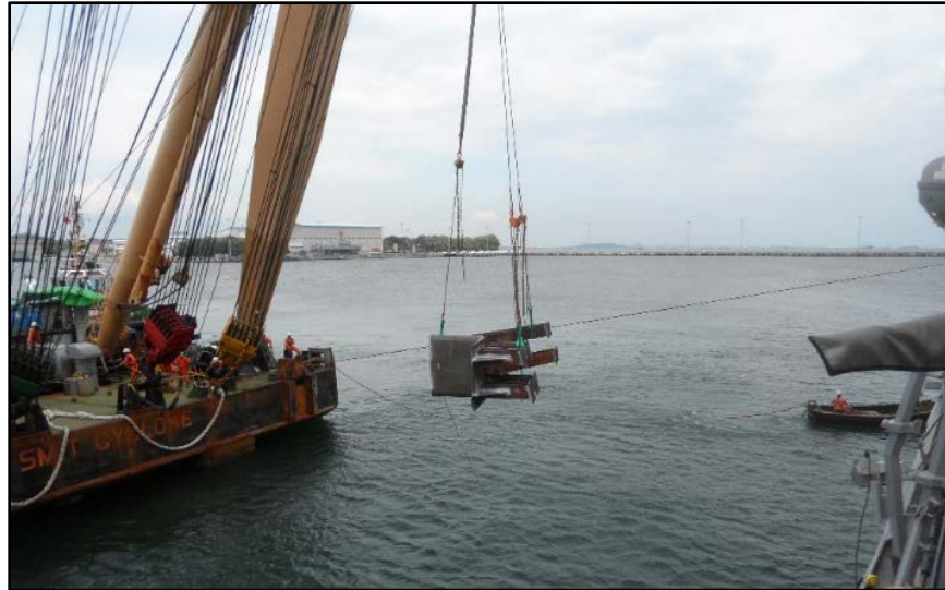
Figure 4-5. Staging the catcher prior to welding onto USS John S McCain
