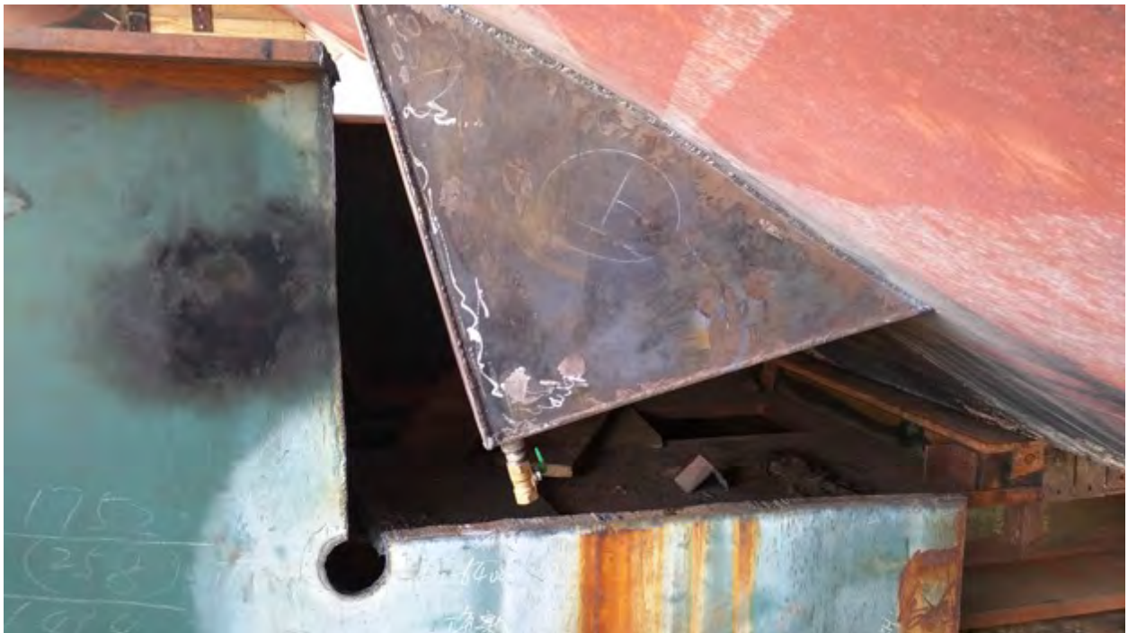
Fig 14. Revised grillage cut on the cargo hull's starboard side.
