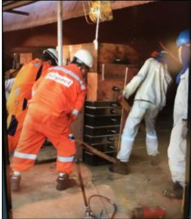
Figure 4-17. Manually positioning block on M/V Treasure
