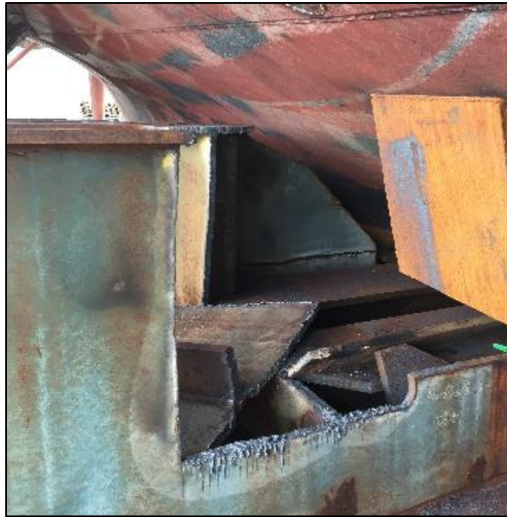
Figure 5-23. Grillage removed prior to offload
