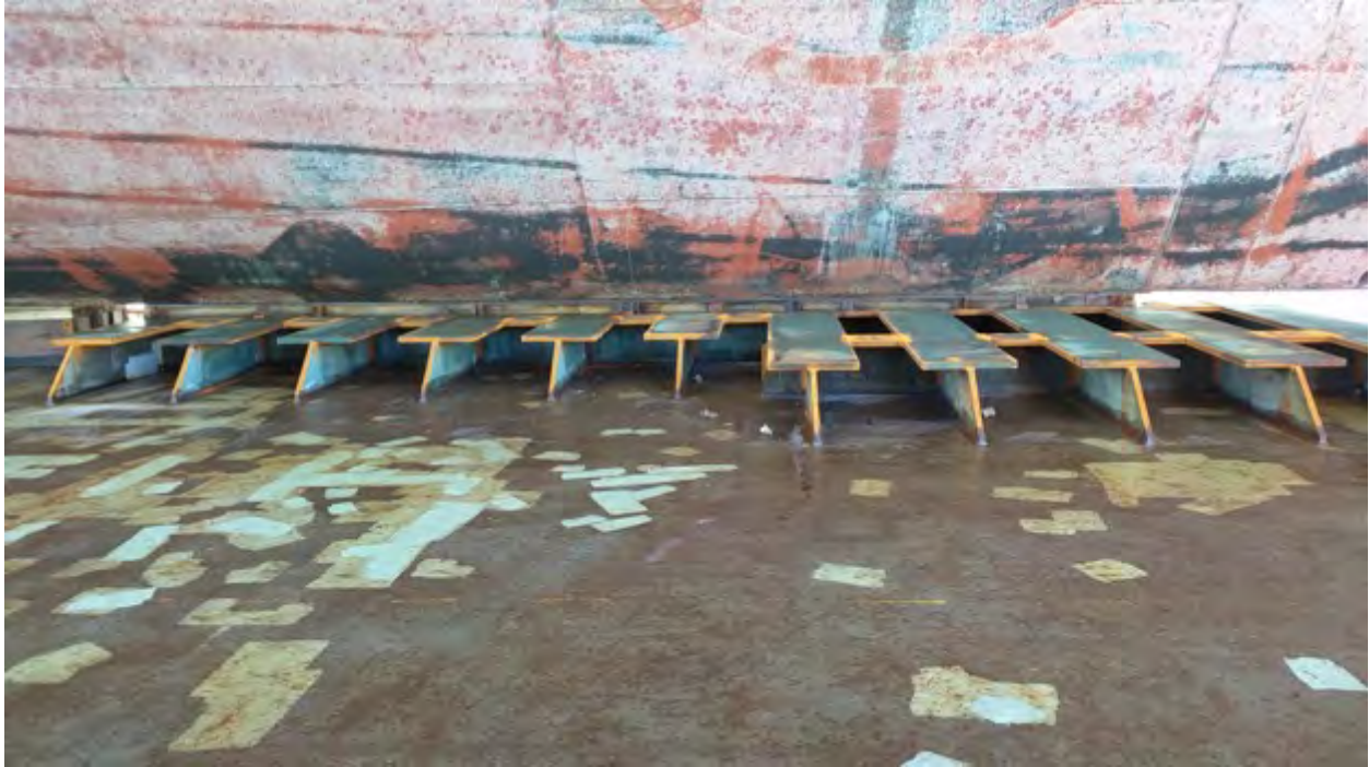
Fig 3. Bow grillage constructed on the cargo deck of the HTV with the cargo in-place prior to installation of sea fastening for transport from SRF Yokosuka.
