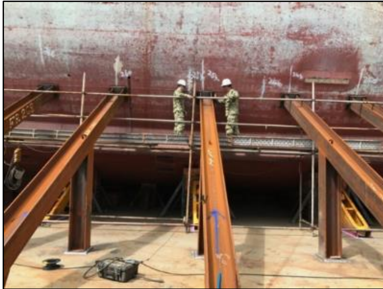
Figure 4-19. Verifying spur shore contact and frame placement
