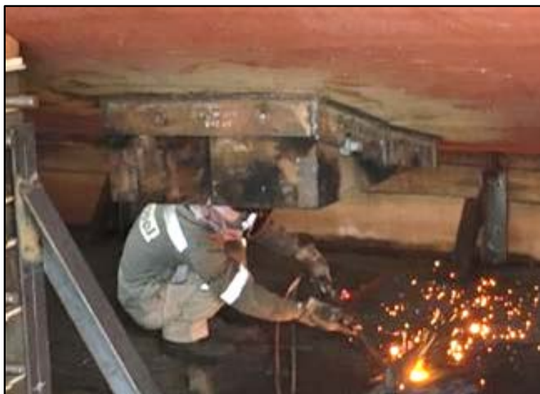
Figure 4-20. Soft cap "DC plugs" under box patches
