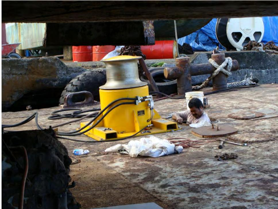
Figure 7. Installation of the ESSM Capstan Aboard the Barge *Derrick*
