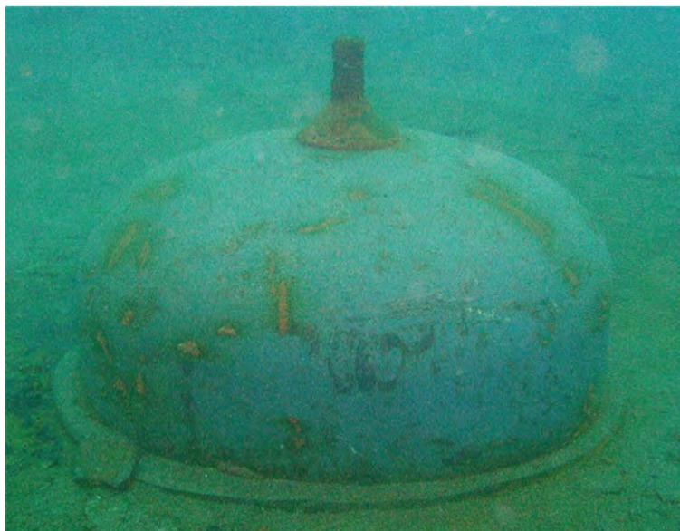
Figure 5-27. Capping the Hot Tap Penetration
