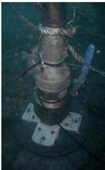
Figure 5-26. Hot Tap Flange Ball Valve and Suction Hose
