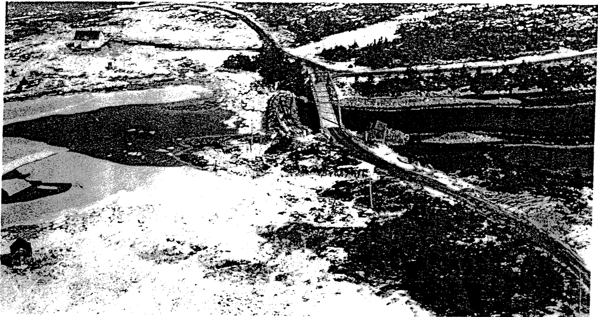
Causeway protecting Canso area against infiltration of Bunker "C" through coastal waterway.
