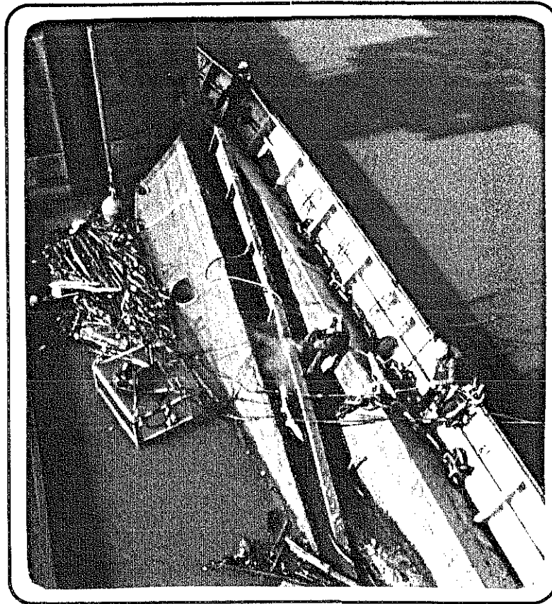
Figure 7.13.1: Diver Deployed in Man Basket to Burn Chain Holes in MST 351
