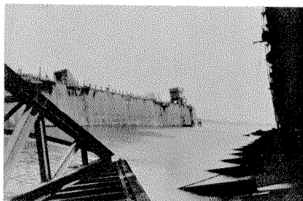
RIISING B WALL shown above surface as drydock rotated to 161 degrees from inverted position.
