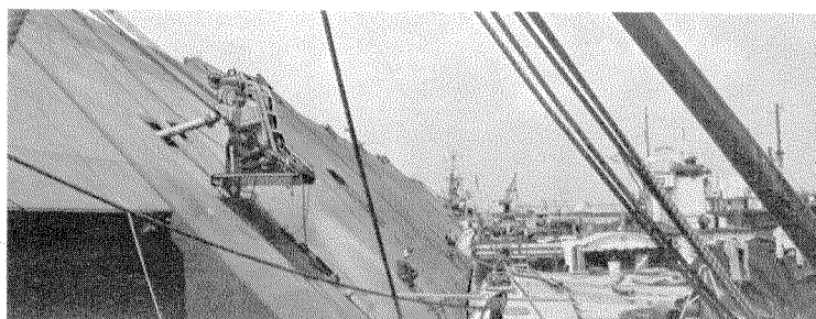
PUMP on platform welded to wingwall was utilized to dewater offshore wall so that inshore side could be grounded on the river bottom.
