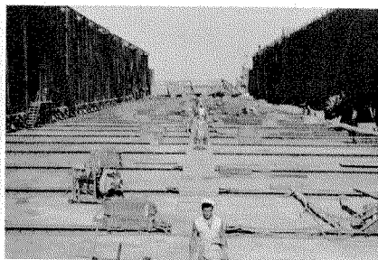
COMPLETELY DEWATERED , AFDM-2 assumed upright position with draft of six feet.
