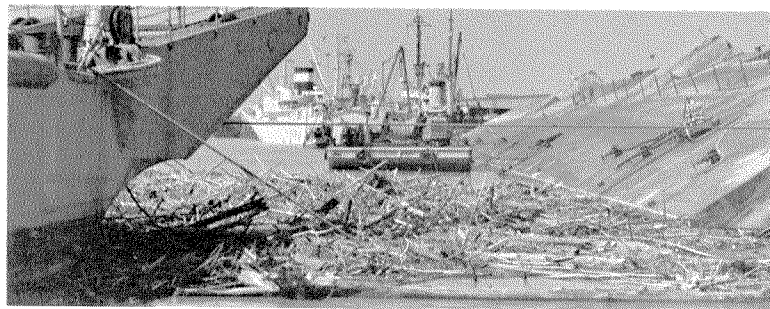
TONS OF DEBRIS , carried by high velocity flood waters, apparently snapped anchor cable of lift ship holding AFDM-2. Drydock was swept to opposite bank of Mississippi River.
