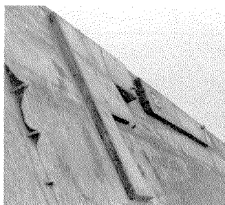
BOX-TYPE steel plates were welded over major breaks in wingwalls.
