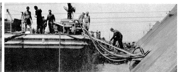
BALLAST was added to inshore compartments of center section. Before drydock would assume Stage I position, 2,000 tons of mud and water had to be removed.
