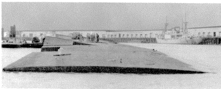
CAPSIZED DRYDOCK'S bottom pontoon sections were not seriously damaged, but more than 100 breaks were found in the wingwalls.
