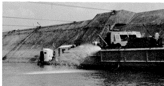
DEWATERING PUMPS, mounted on work barges, removed ballast as beach gear continued to exert pull.
