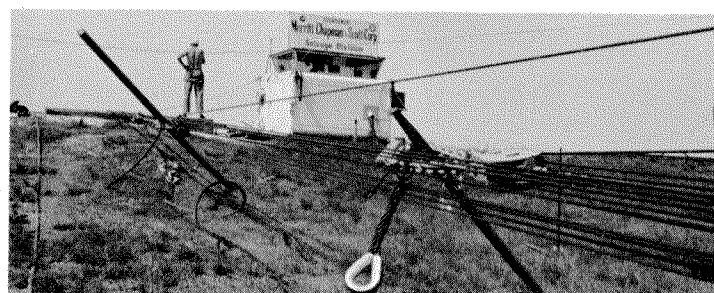
CONTROL CENTER housed stylus recorders that indicated beach gear force. From this central location engineers were able to control rate of pull.
