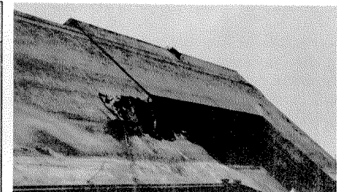
BIGGEST BREAK was an oval-shaped gash, 20 feet by 15 feet, at the end of the center section.
