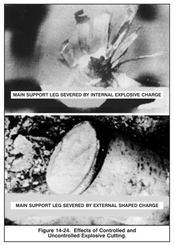
**14-6.3** <u>Charge Placement</u>. Weight and placement of underwater explosive cutting charges must be planned to:
