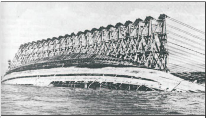
Figure 7-15. Braced-Girder Headframes on USS OKLAHOMA.
