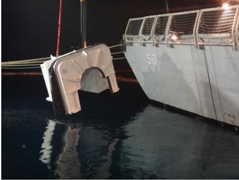
Hub cofferdam being lowered into the water for a test fit.
