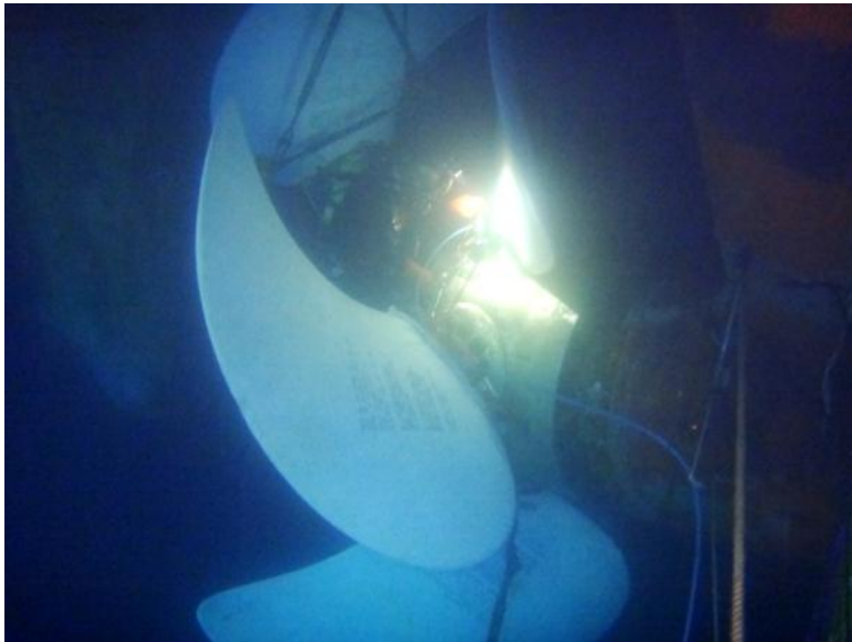
8 April 2014 image of new hub with the blade installation in progress.
