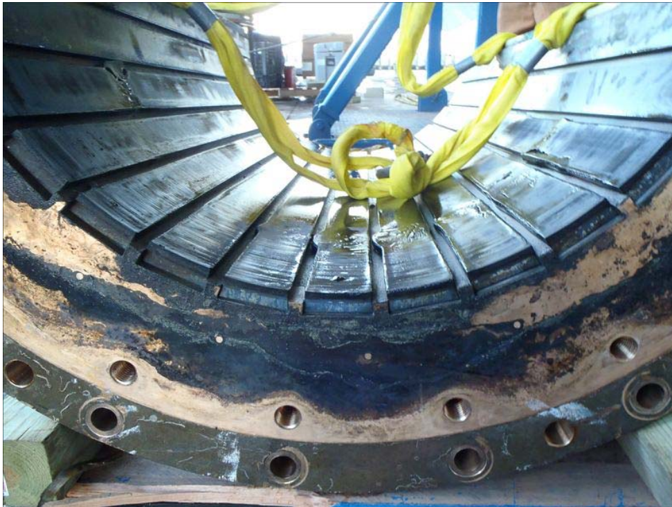
Damaged staves are visible on the bottom half of the stern tube bearing. This bearing is resting on the dive and rigging barge prior to being transferred to NNSY's bearing shop.
