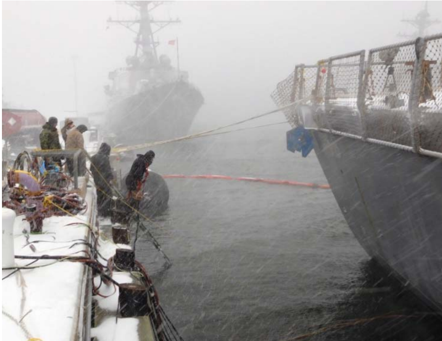
SUPSALV's contract welder/diver enters the water to reach the underwater habitat which allowed for dry welding on USS LABOON's rudder.
