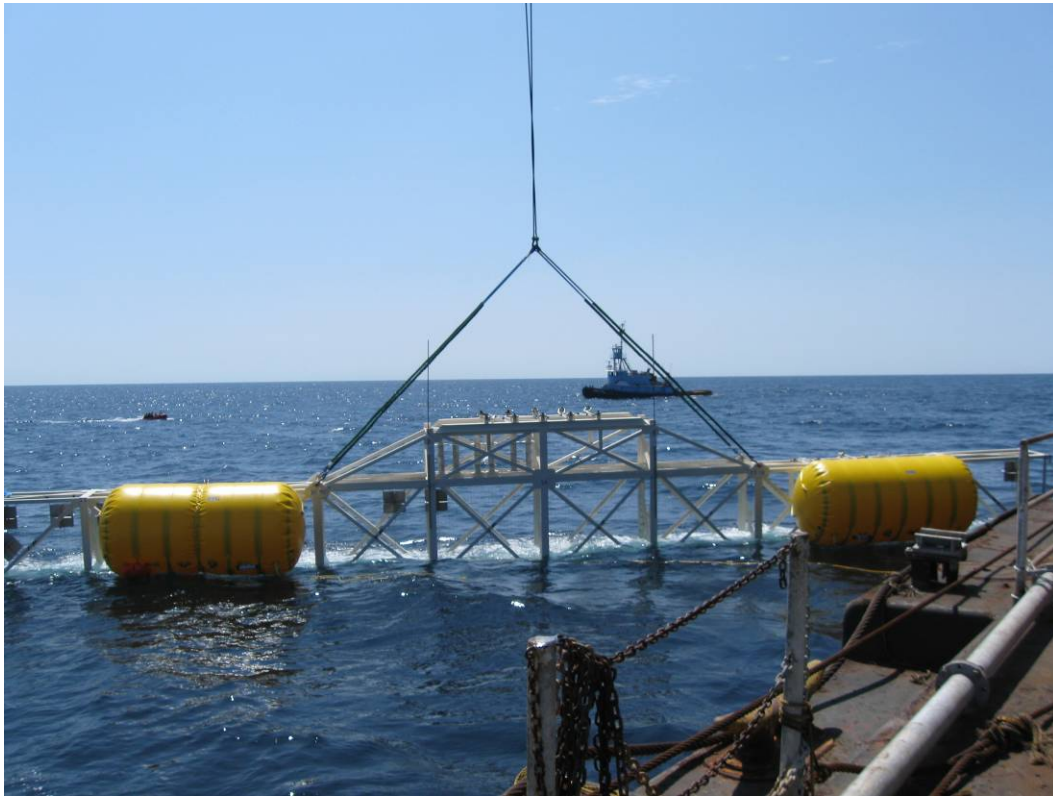
One of the targets being lowered into the water. The yellow air bags will keep the target floating near the surface. DONJON's tug Mary Alice is in the background.
