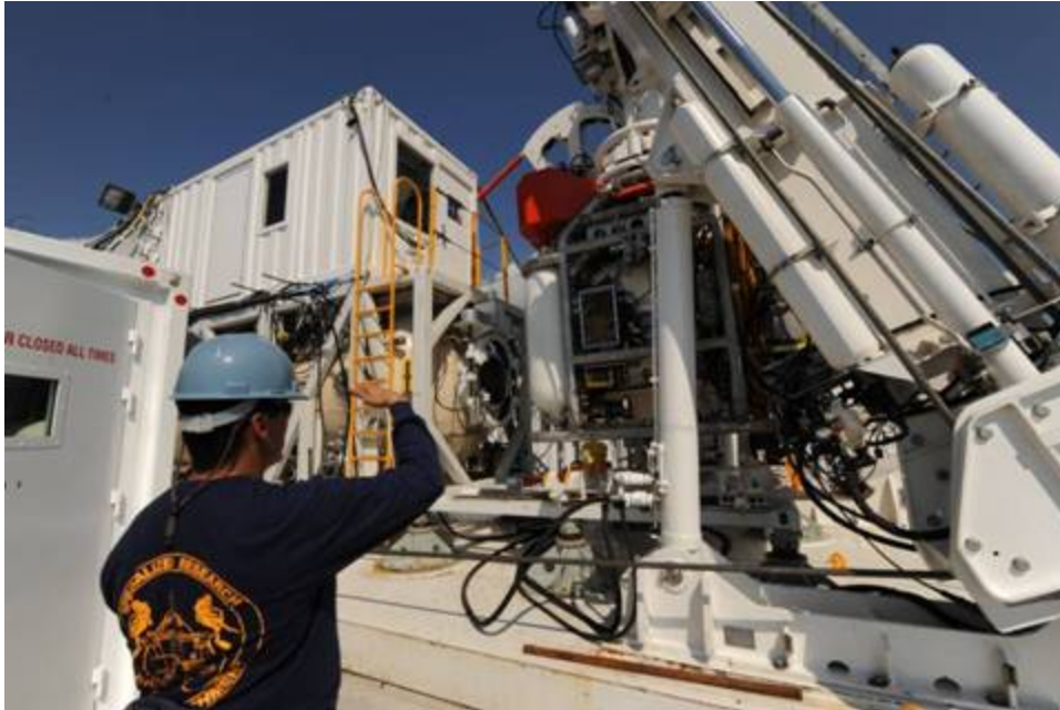
Components of the SAT FADS system on the pier at NEDU. Bell handling system to the right and living quarters underneath the control van on the left.
