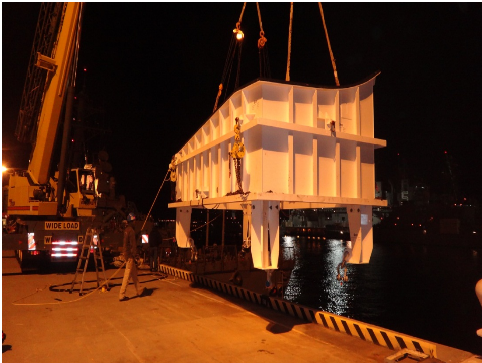
One section of the new three-piece rudder cofferdam being moved from the pier to the water for fitting onto USS MAHAN (DDG 72).
