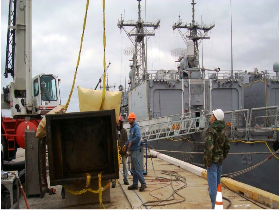
An image of the traditional 4' x 4' dry habitat being rigged for use.
