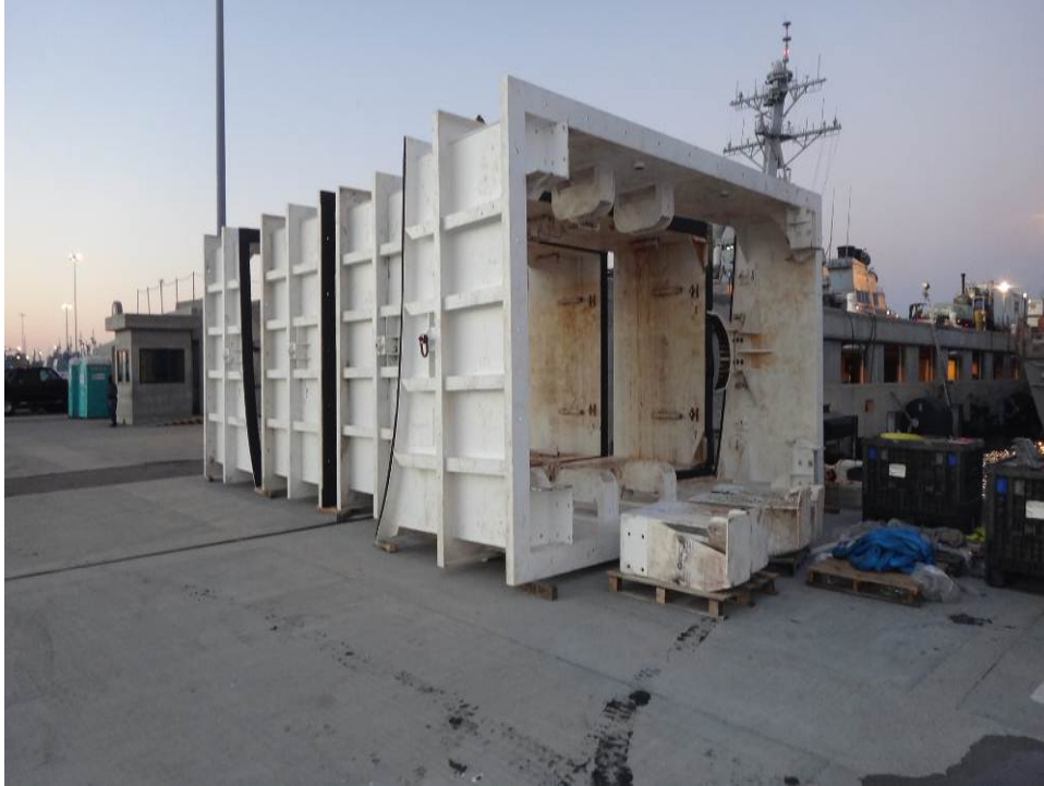
The three sections of the full cofferdam are shown on Pier 6 in Norfolk Naval Station.
