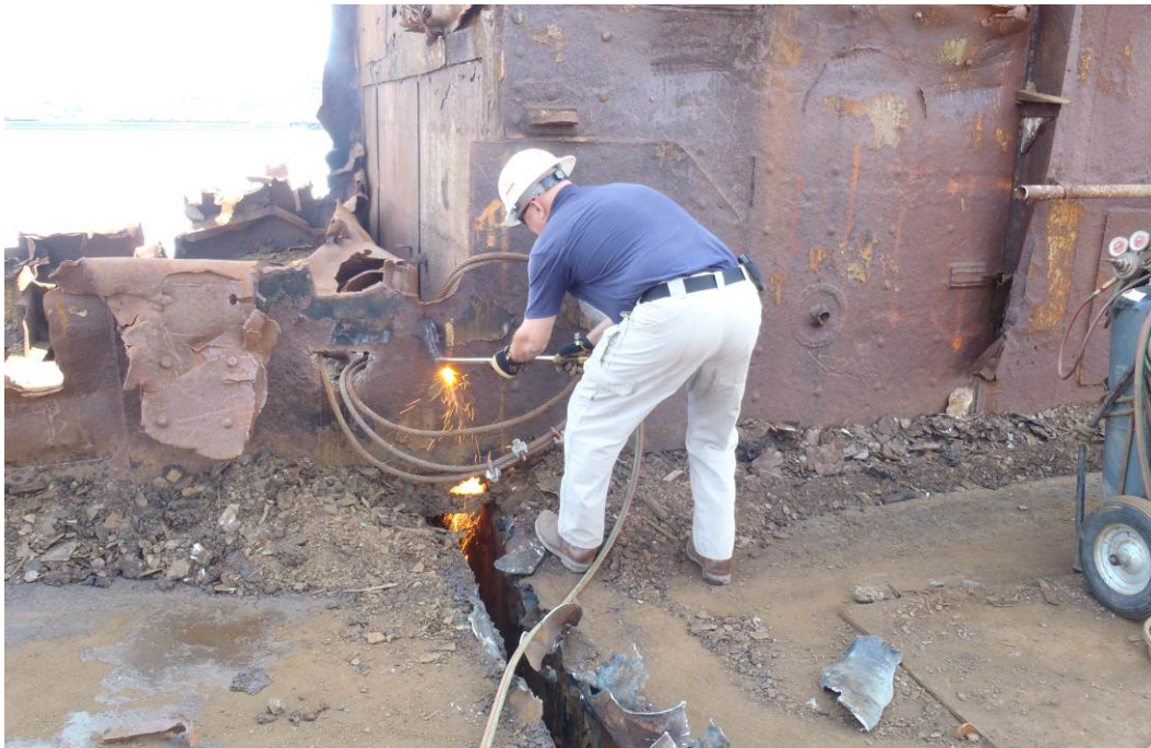
SUPSALV Representative makes final cut to disconnect the aft end section.
