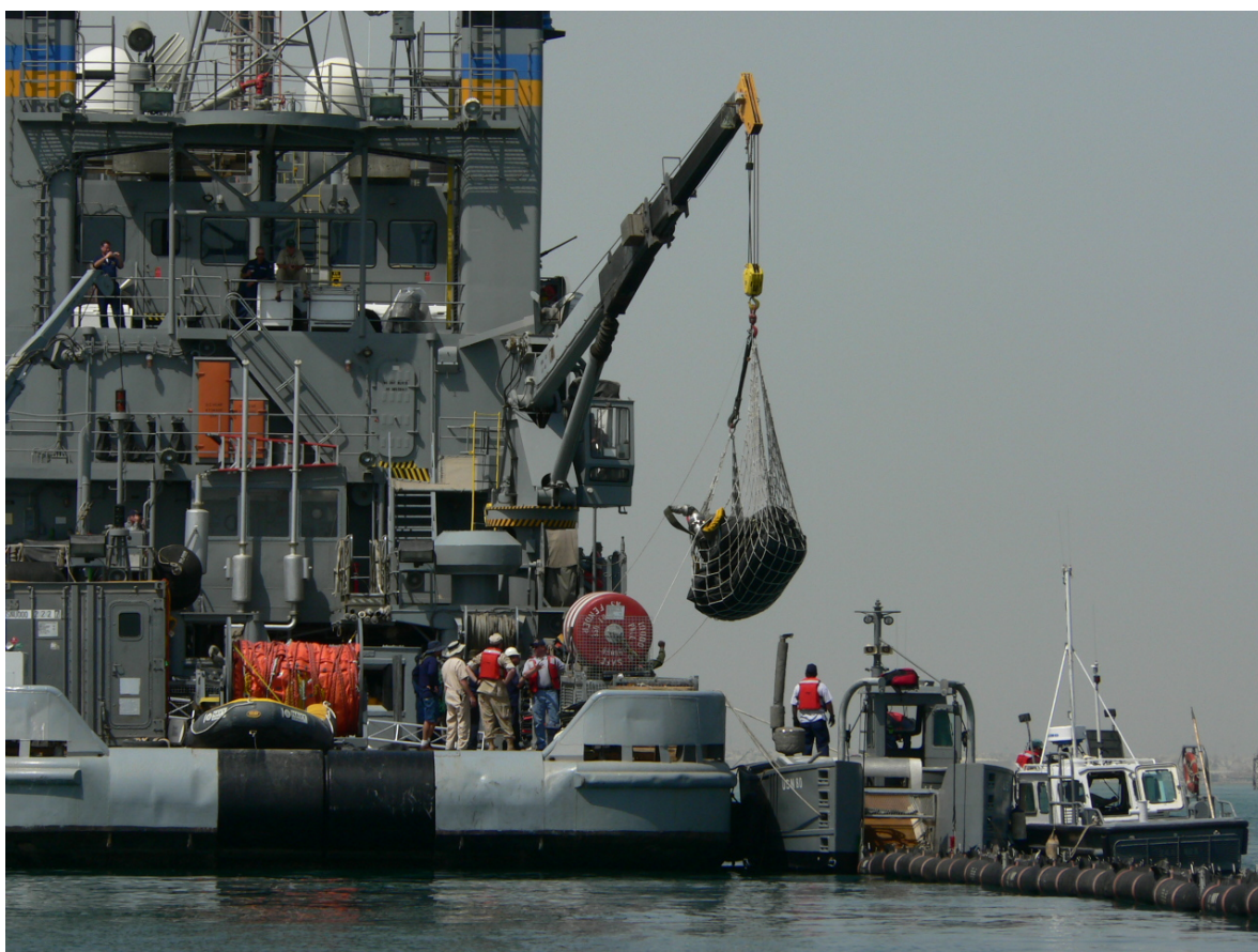
Figure 10-48. Deploying the Oil Recovery Bladder
