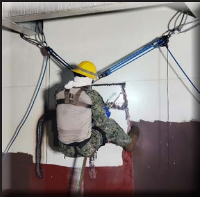
Navy Diver from Mobile Diving and Salvage Unit ONE conduct exothermic cutting and rope suspension for Battle Damage Repair/Assessment training.
