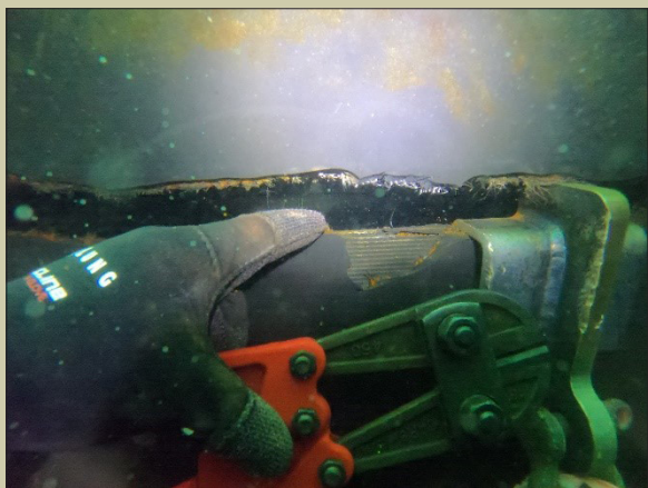
Upper and Lower SDRW alignment in progress with ruptured edge grooming.
