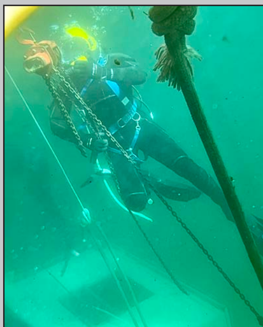
ND2 Craffey righting the tug using a chain fall.
