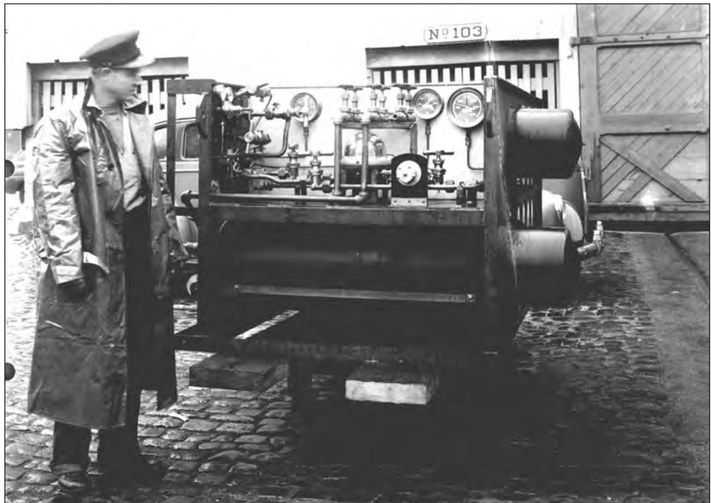
**Figure 1-14.** Helium-Oxygen Diving Manifold.
