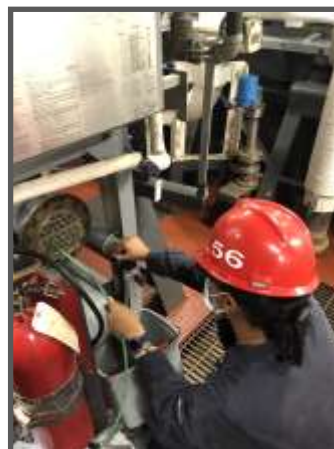
MM1(SW) Patrice Braswell from Lawton, Okla., cleans the condenser tubes of number one reefer with a hydro lance aboard USS Port Royal (CG 73). MM1 has earned three (3) NECs while at Pearl Harbor: Air Conditioning and Refrigeration Repair Technician, Watertight Closure Maintenance Technician, and Valve Repair Technician. (Photo by MM1(SW/AW) James Weierbach.)
