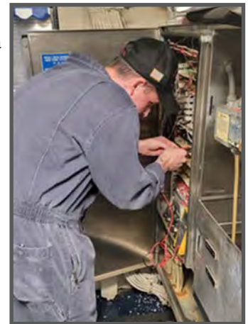
EM3 Kaleb Stryd from USS New Orleans (LPD 18) taking readings on relays for the Gaylord Vent System Washdown. (Photo by Rizalito Antonio.)
