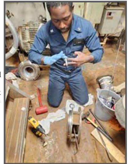
MM2 Armstrong Calixte from Port Au Prince, Haiti lubricates the mechanical seal cartridge prior installation on Nr.4 Chill Water Pump.
