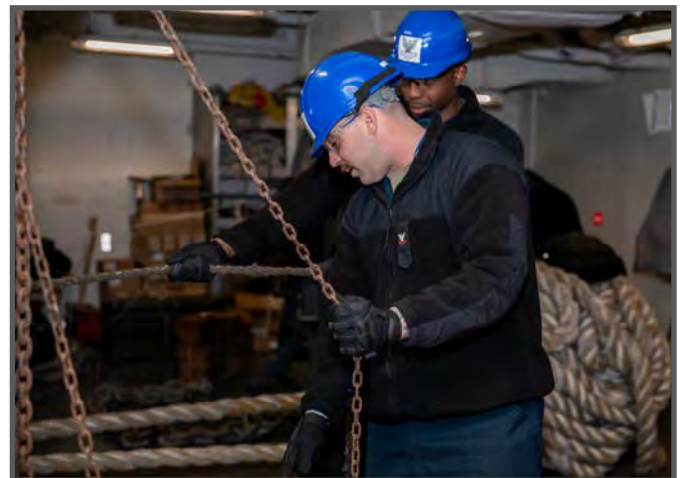
BM2 Donald Williams and BM2 Robert Swanson discuss safety and rigging strategy to remove a 900 lb plate as part of the NAMTS Rigger/Weight Tester JQR to earn the associated Navy Enlisted Classification (797A). (Photo by USS George H.W. Bush Public Affairs.)
