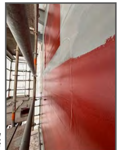
Patches were sealed and primed. Ship's force will apply the topcoat to match the area.
