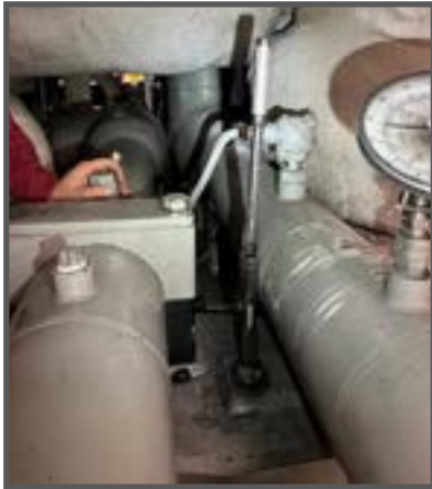
The unique way MR2 (SW/AW) Gabriel Donovan came up with to re-tap each of the foundation holes.
