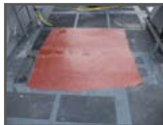
Patch with the polysulfide sealer and primer applied.
