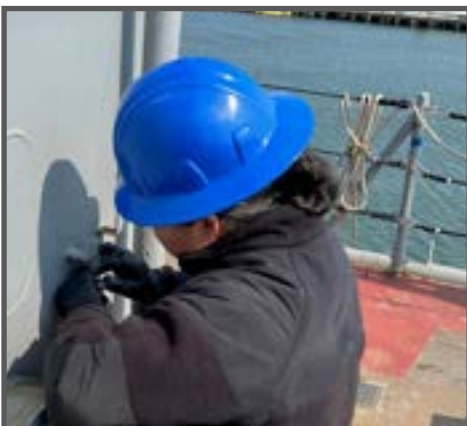
Seaman Mariana Martinez of Salem, Ore., applies Sailor Putty to a corroded bracket on USS Tortuga (LSD 46) on May 18, 2023. (Photo by Kat Ciesielski, NAMTS Public Affairs.)
