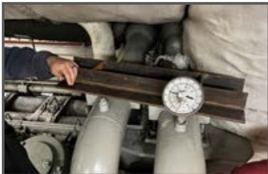
The exoskeleton framework that HT2(SW) Joshua Smutzer and HT3(SW) Jesus Aranda custom made for retaining the main engine cooling pipes.
