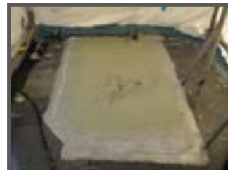
Manually sand the cured patch area in preparation for the polysulfide sealer.
