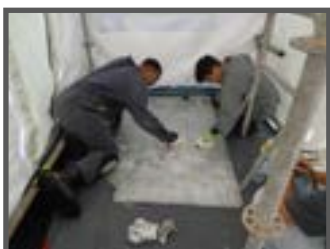
Scrubbing the surface ensuring no debris is present prior to applying pre-resin treatment.
