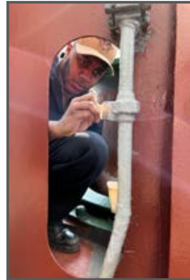
USS Tortuga's (LSD 46) PS3 Rodrec Person of Ocean Springs, Miss., wrapped a pipe in S2S Sailor Putty then painted over it using the paint cartridge system and polysiloxane paint on May 18, 2023.
