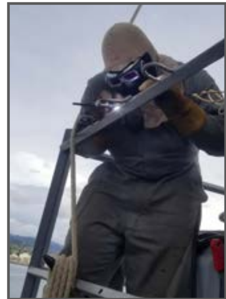
HT2 Patrick Johnson conducts a welding job on a signal shack life rail aboard a DDG. (Photo by HTC London Hunter.)
