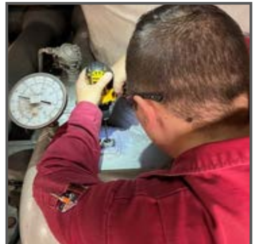
MR2(SW/AW) Gabriel Donovan drilling into a piece of broken bolt in one of the piping foundations.
