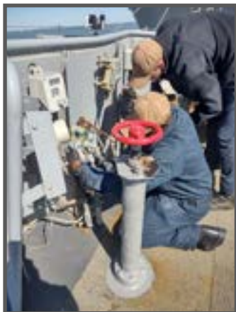
USS McFaul (DDG 74) Sailors apply a one step anti-corrosion tape called "Sailor putty" to piping.
