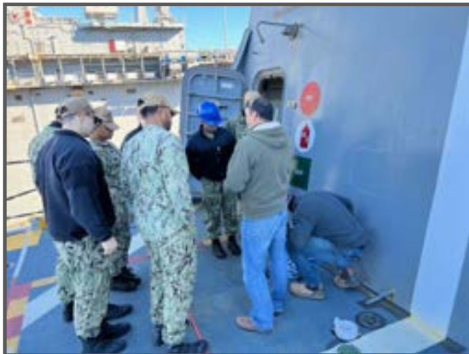
Ship 2 Shore, Inc. representatives conduct a demonstration of the application of Mil-Spec material on bulkhead corrosion areas on October 20, 2022, aboard USS New York (LPD 21).
