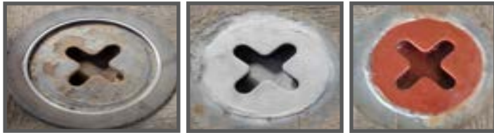
Left: A cloverleaf tiedown with visible corrosion before being blasted Middle: Blasting results in an SP-10 finish Right: The tiedown is primed and preserved (Photos by Andy Vasquez.)
