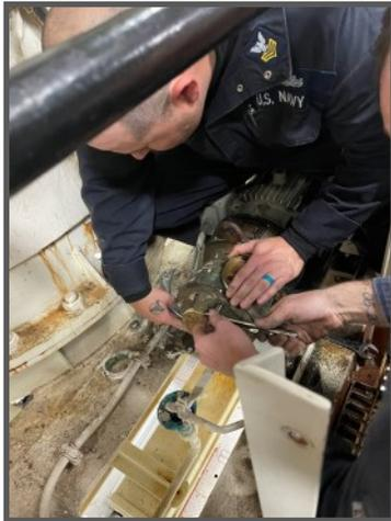
MM1(SW) Jonathan Silva replaces a mechanical seal on a hot water recirculating pump aboard USS Jason Dunham (DDG 109). (Photo by MMC(SW) Gordon Reichert.)
