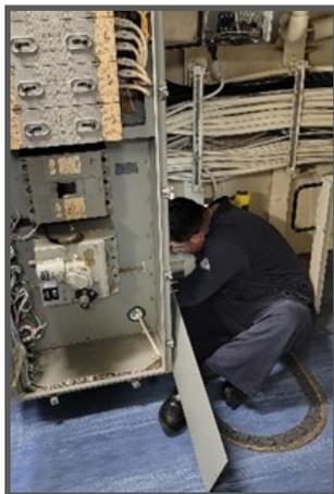
Left: EM2(SW) Oscar Alfaro seen above is taking resistance readings on the transformers inside the 400 HZ switchboard as part of the troubleshooting of the ground indicators for the 400HZ switchboard. (Photo by Rizalito "Tony" Antonio.)
