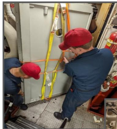
USS Stethem's DCFN William Nadler (left) and DC3 Nathan Harris position the balanced joiner door in preparation for installation. (Photo by LTJG Bryant Chau).
