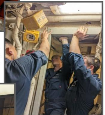
Left: DCFN Rikardus Bowano (center) and DC3 Nathan Harris (right) centering the Balance Joiner Door Frame into the ship's bulkhead. (Photo by LTJG Bryant Chau).
