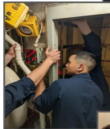
Right: DCFN Samuel Caruso installing the Balance Joiner Door frame bolts into the ship's bulkhead. (Photo by LTJG Bryant Chau).
