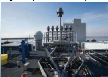
Satellite Communications Deck
