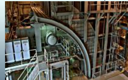
Advanced Submarine Launcher Facility
