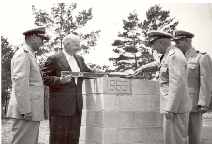
The centerpiece of the 10th Anniversary celebration was the laying of the cornerstone for the new main building (Building 110). - The Underseer , July 1955
