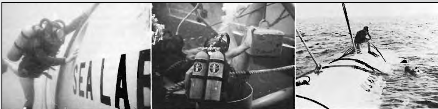
These photos, taken by the Navy Mobile Photo Unit from Norfolk, Va., depict the precarious work necessary to prepare the SEALAB I experimental, underwater habitat for its big test in Bermuda in July 1964. (left) Gunners Mate First Class Lester Anderson, one of the Navy men who would live in the SEALAB I during the Bermuda test, makes external checks while SEALAB I was resting on the bottom of the Gulf of Mexico in Panama City, Fla. (center) One of the Navy divers from the YFNB-12 vessel guides ballast weights into the bins of SEALAB I, which was one of the real precarious missions performed undersea. (right) Navy divers check the secure lines and other apparatus as the YFNB-12 prepares to lower SEALAB I to the seabed. SEALAB I, designed and built here at MDL, would depart for Bermuda aboard the YFNB-12 in early June 1964.
