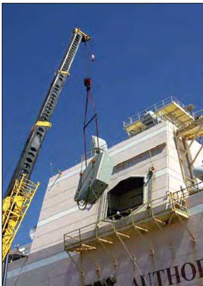
Figure 5. SPY-1A Array Being Uninstalled from the SWEF
