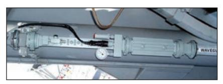
Figure 2. Sulfur Hexafluoride (SF6) Gas-Filled Filter Installed Aboard USS Tarawa
