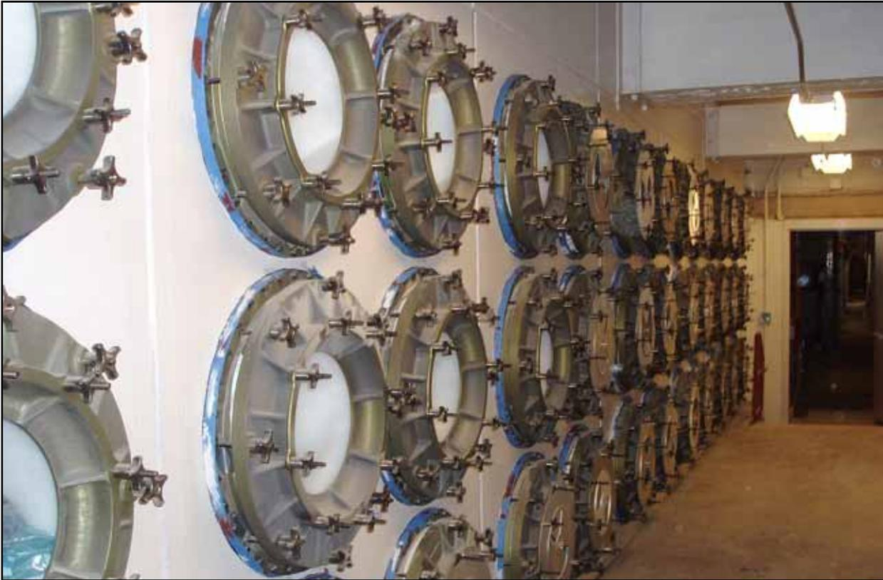
**Figure 2.** CBR Collective Protection Filter Housings Installed in a Facility
