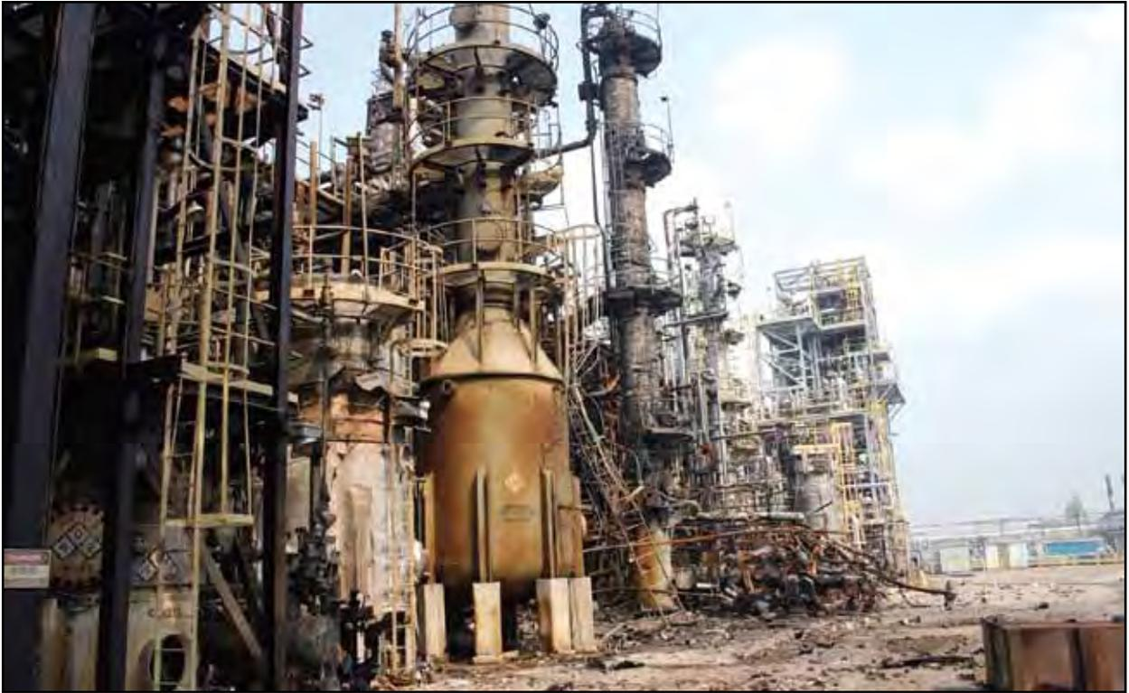
**Figure 1.** Two workers were fatally injured when a waste tank containing the pesticide methomyl violently exploded, damaging a process unit at the Bayer CropScience Chemical Plant in Institute, West Virginia.<sup>1</sup>
