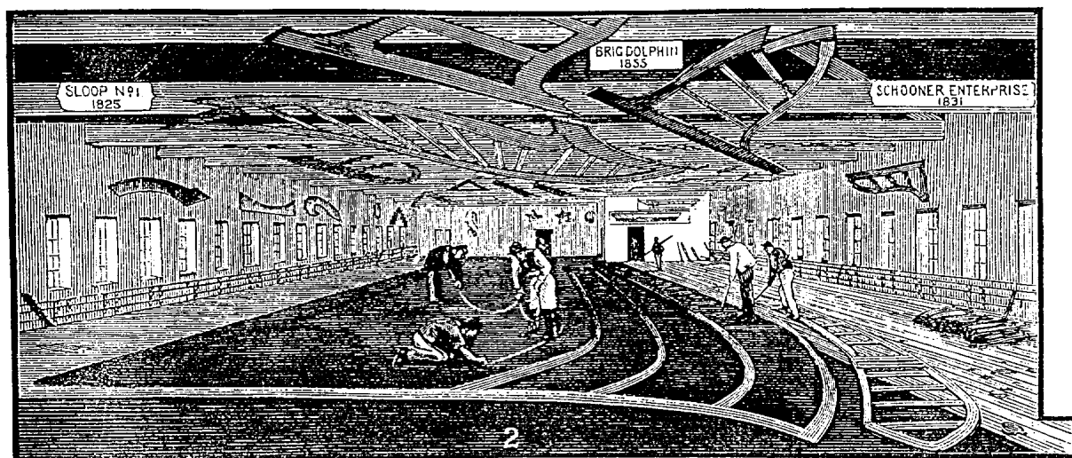
Loftsmen laying off the battleship Maine , New York Navy Yard, 1889. The kneeling worker in the foreground is holding the end of a batten that will be used to scribe a sweeping line on the floor. Nearby, two figures adjust a measuring tape. Ceiling joists are adorned with plaques commemorating previous designs laid off in the loft. ("Sloop No. 1" became USS Lexington .) Sturdy moulds are stored overhead. Two old half models are mounted on the far bulkhead. Harper's Weekly , March 9, 1889.
