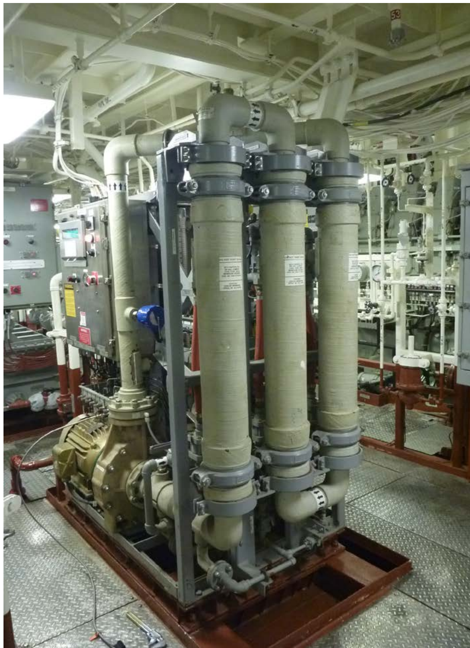
Shown above, the oily waste processing systems currently installed on USS Arlington (LPD 24). It uses three ceramic membranes to process the wastewater. The costs, as well as the fragile nature of the membranes, drive the need for a procedure that does not require filter disassembly. (U.S. Navy photo by Syed Shamim/Released)
